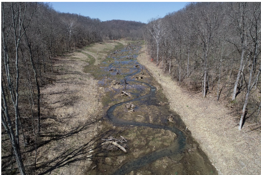
Drone photo of Beham Run, which is an approximately 8,000 LF reach of floodplain restoration with about a 10-mile drainage area. This picture was taken at the start
