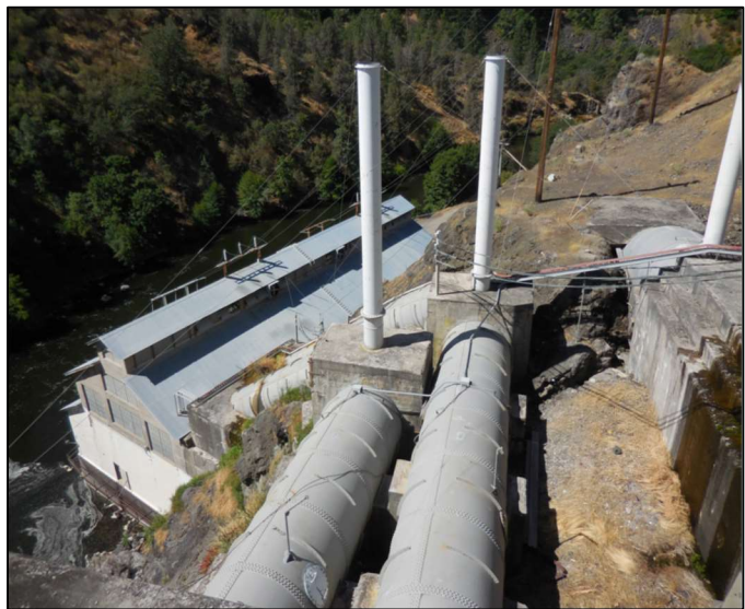
PHOTO 7 COPCO No. 1 10-FT (LEFT AND MIDDLE) 414-FT (RIGHT) PENSTOCKS
