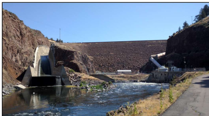
PHOTO 14 IRON GATE DAM, SPILLWAY (LEFT), AND POWERHOUSE (RIGHT)
