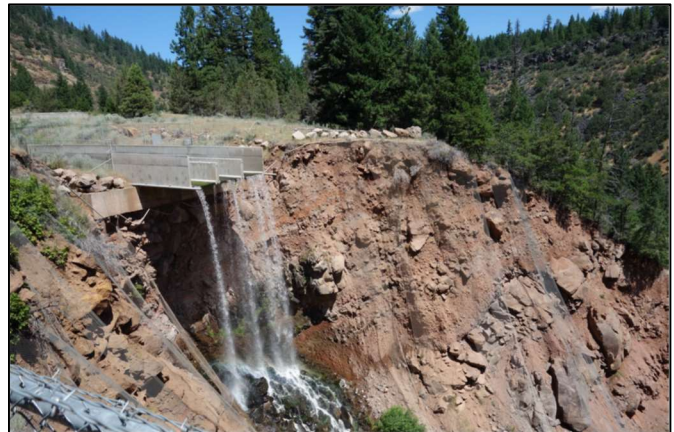
PHOTO 4 J.C. BOYLE FOREBAY OVERFLOW CHUTE AND UPPER PORTION OF SCOUR HOLE
