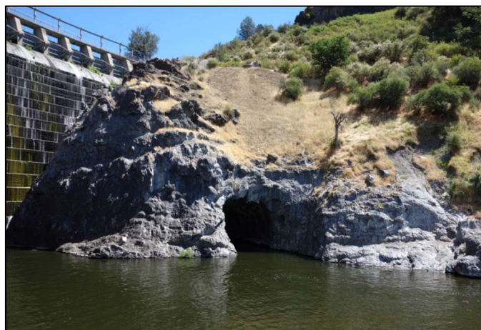
PHOTO 6 COPCO No. 1 DIVERSION TUNNEL DOWNSTREAM PORTAL
