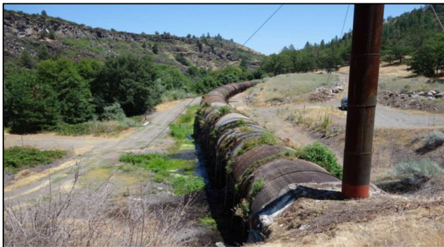
PHOTO 11 COPCO NO. 2 WOOD-STAVE PENSTOCK
