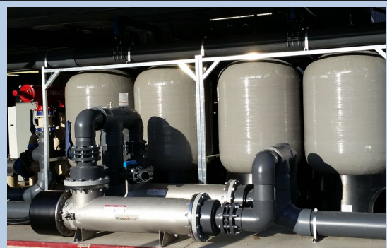
Water Filtration System at Iron Gate Hatchery
