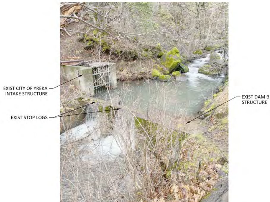
Figure 3. Dam "B" Intake Photograph
