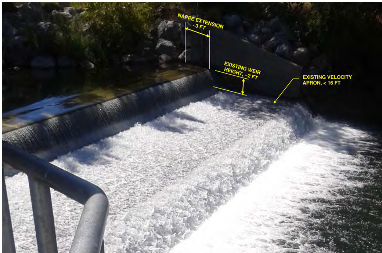
Figure 3-11. Nappe Extension Retrofit (Source; McMillen Jacobs)
