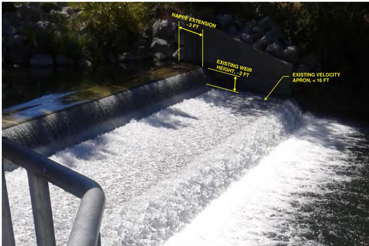
Figure 3-8. Nappe Extension Retrofit (Source; McMillen Jacobs)
