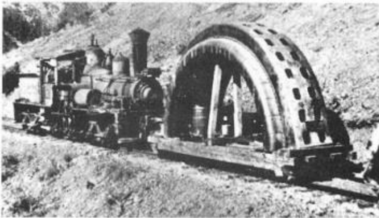
Figure 5-10 The KLRR in 1922, moving part of a generator field down the spur switchbacks to the Copco No. 1 powerhouse
