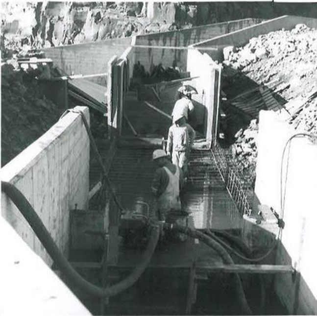
Figure 5-24 Iron Gate dam fish facilities, fish ladder construction, December 27, 1961 (PacifiCorp archive image IG-231)
