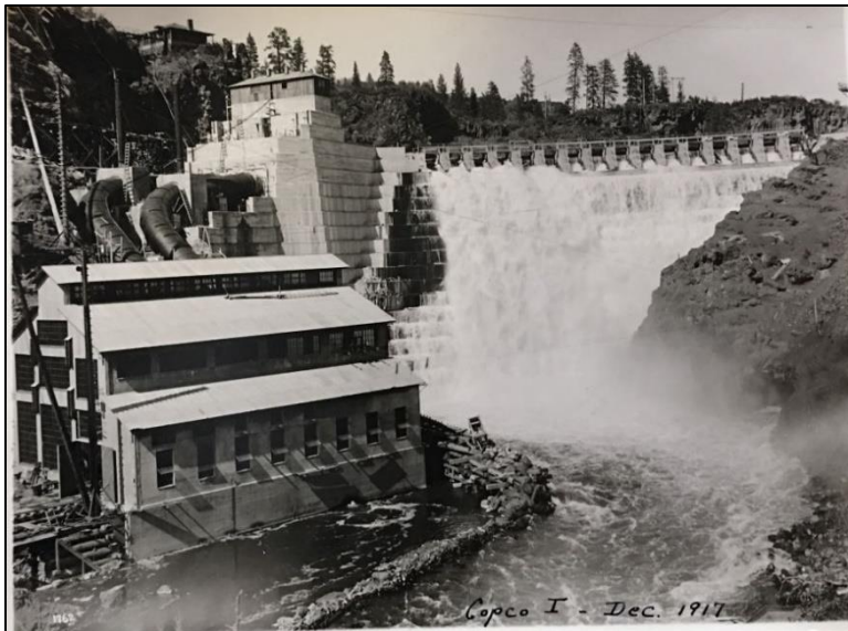
Figure 5-14 Copco No. 1, showing powerhouse, dam, and gatehouse no. 1, December 1917 (courtesy of the John C. Boyle Collection, Southern Oregon Historical Society)
