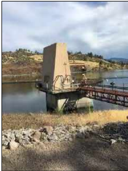
Photograph 5-3: Penstock Intake, Iron Gate
