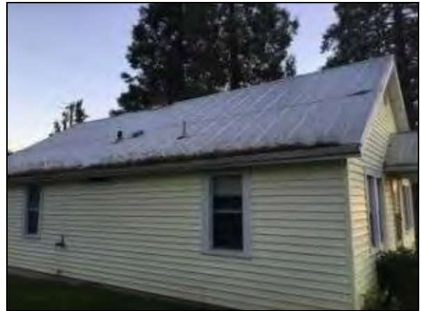
Photograph 5-2: Vacant House #21601, Copco Access Road
