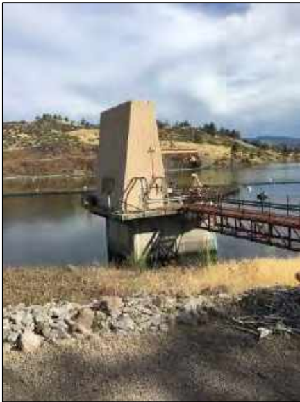
Photograph 5-3: Penstock Intake, Iron Gate
