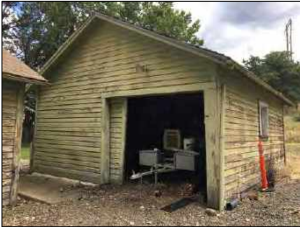
Photograph 5-1: Garage of Vacant House 3, Copco Village
