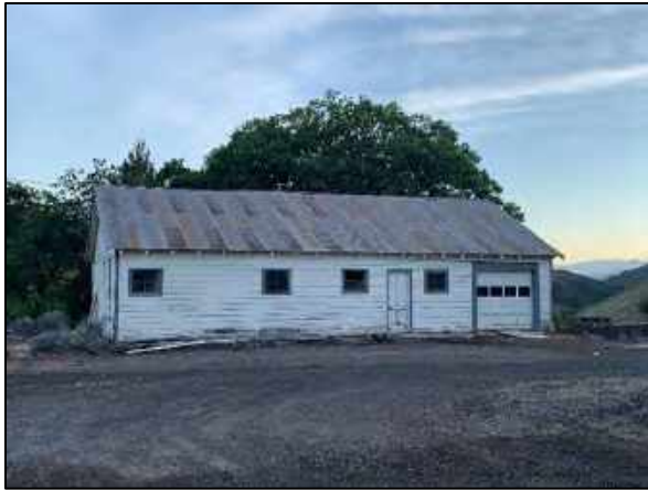
Photograph 3-1 Maintenance Building on Copco Access Road, June 15, 2019
