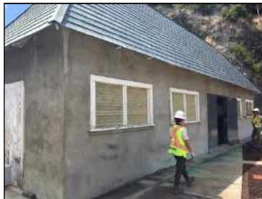
Photograph 5-5: C-12 Gatehouse, Copco No. 1
