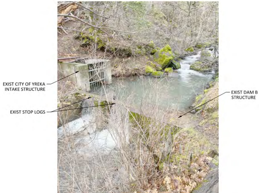
Figure 3. Dam "B" Intake Photograph
