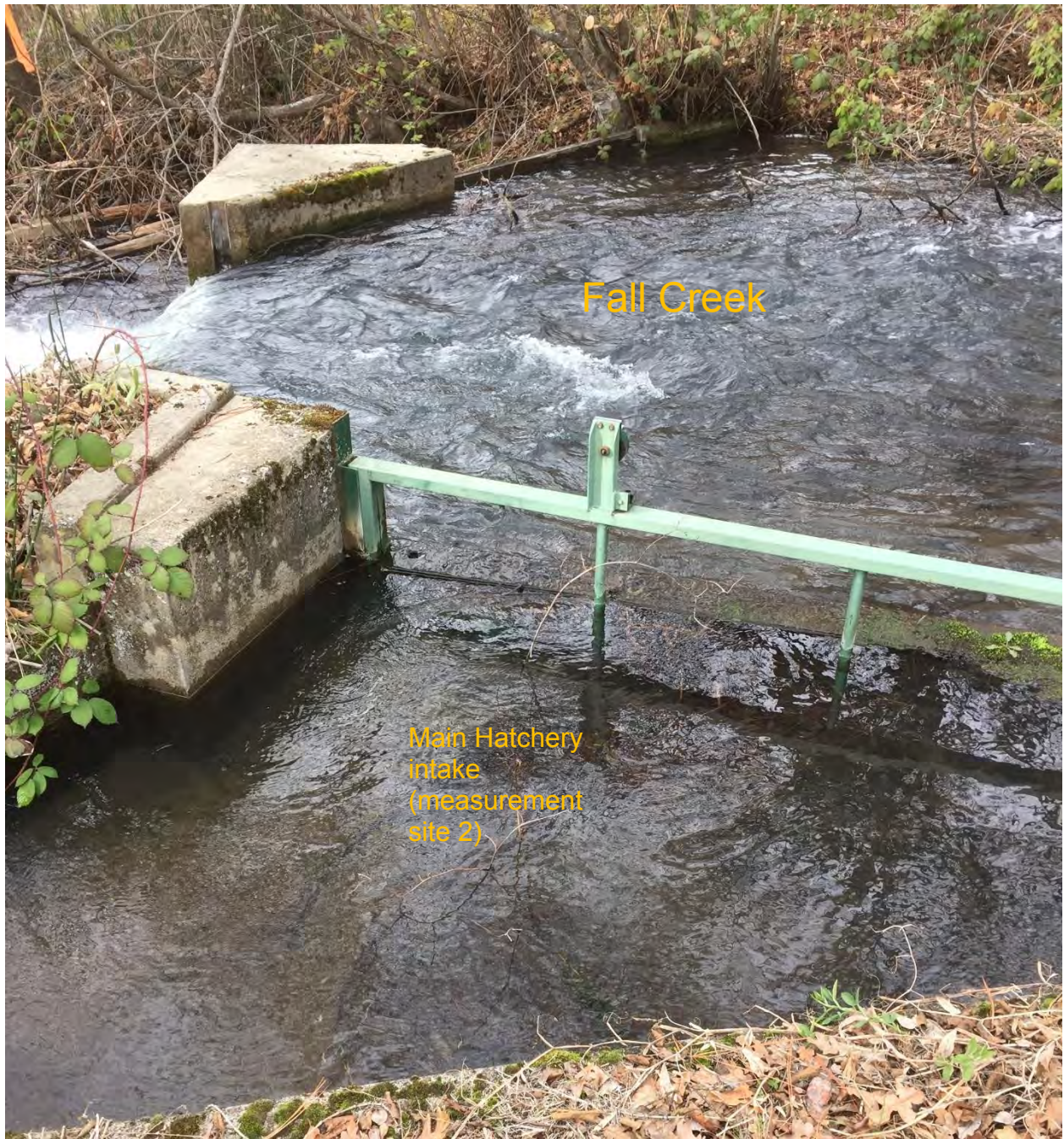
Picture 4: Hatchery intake from Fall Creek below Dam B
