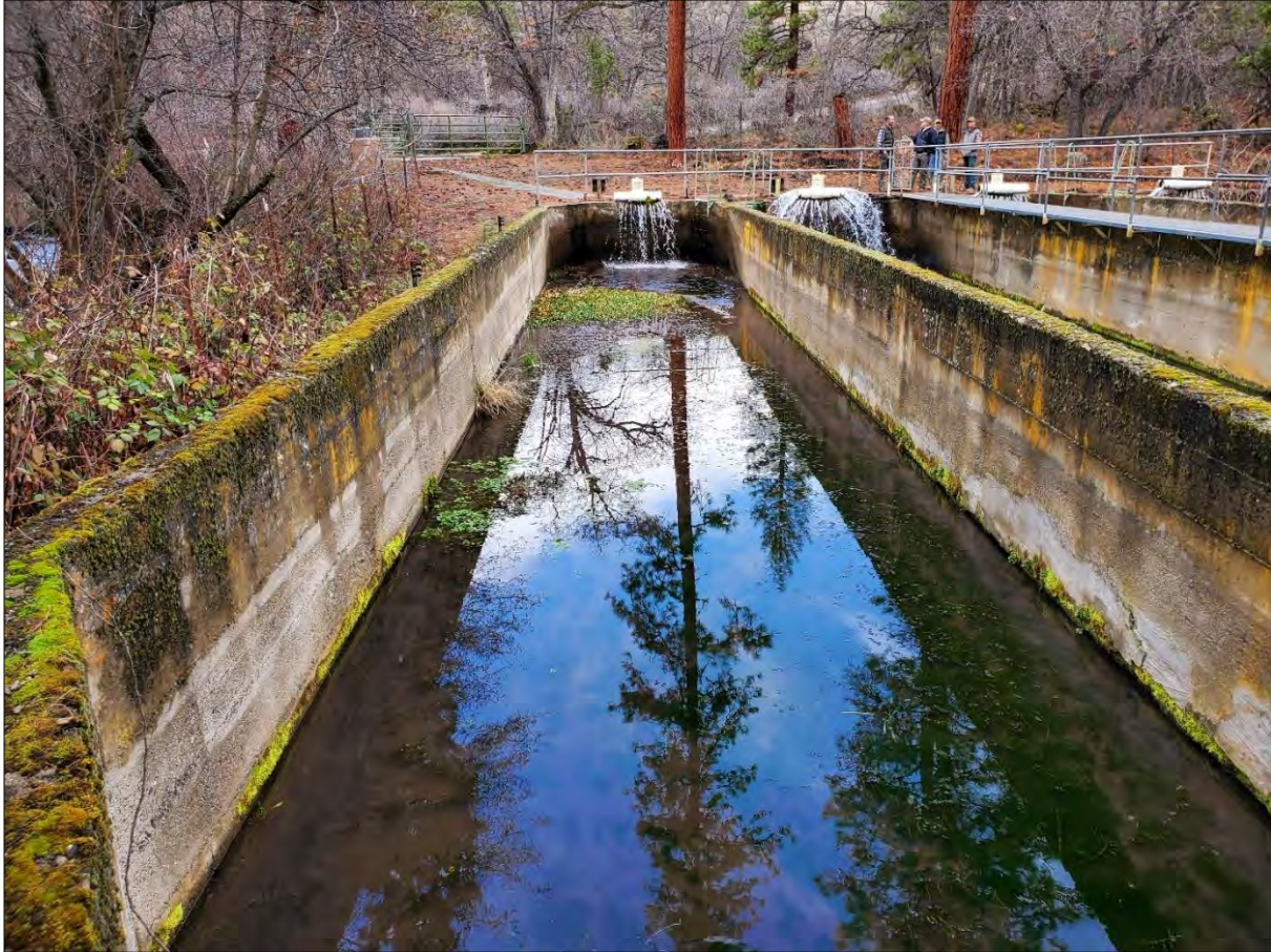
Figure 3-5. Existing Lower Raceway Bank Ponds (Source: McMillen Jacobs)
