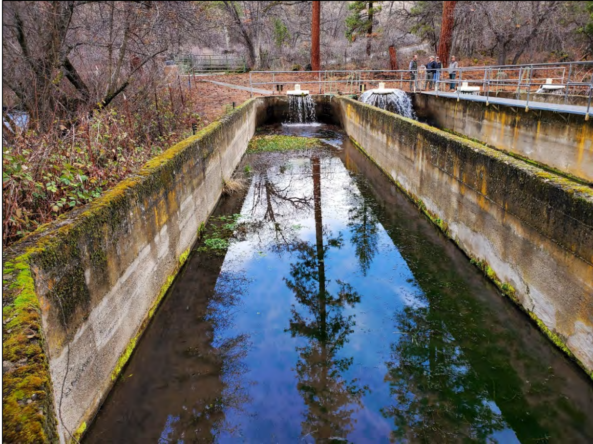
Figure 3-8. Existing Lower Raceway Bank Ponds (Source: McMillen Jacobs)
