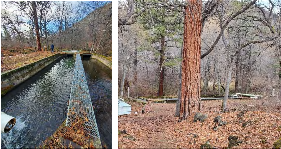
Figure 3-4. Existing Upper Raceway Bank (Source: McMillen Jacobs)
