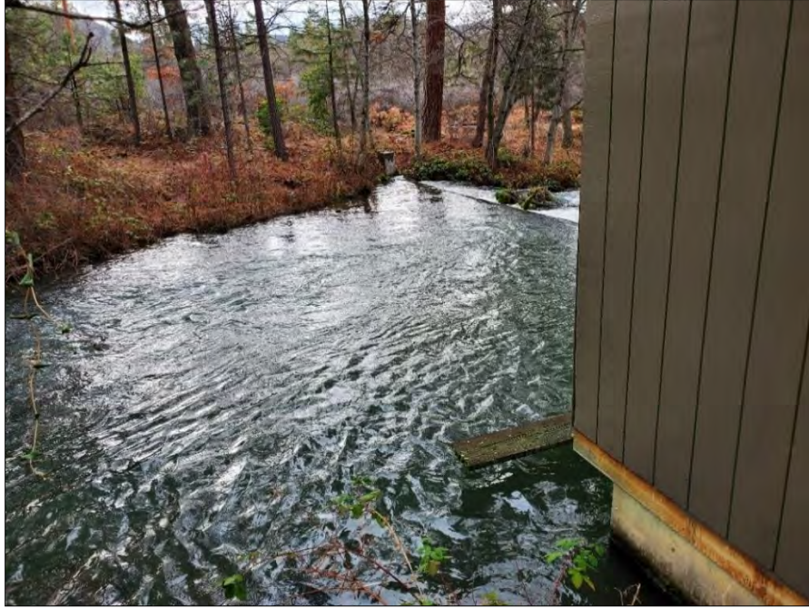
Figure 3-1. Intake Structure Location and City of Yreka Intake (Source: McMillen Jacobs)
