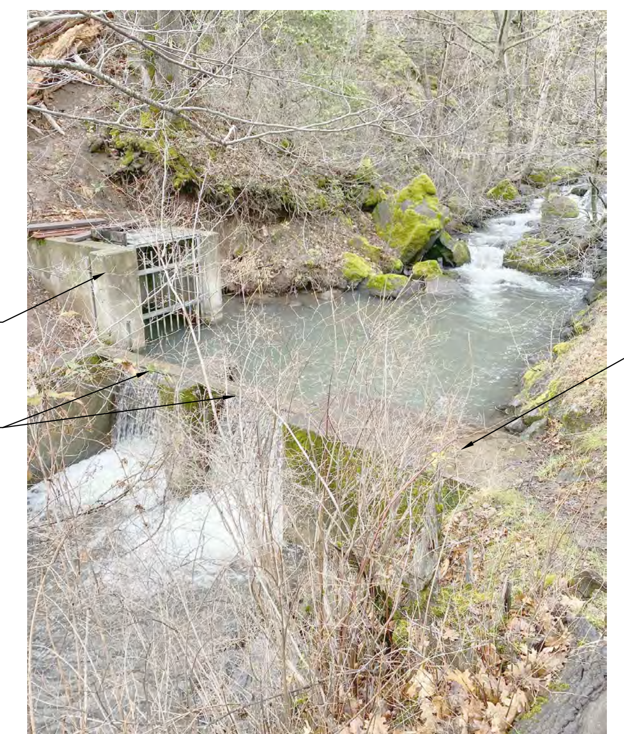
EXISTING DAM B PHOTOGRAPH SCALE: NTS
