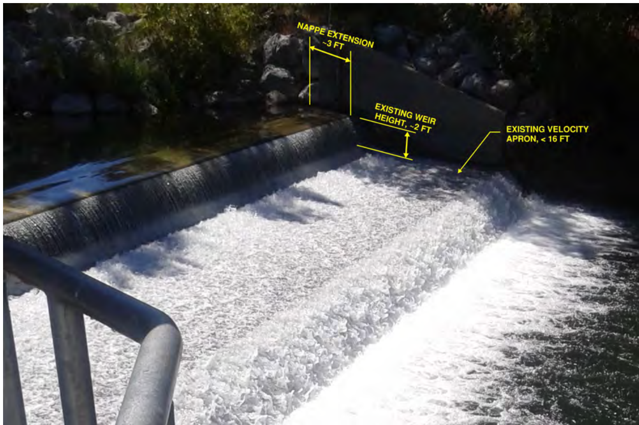
Figure 3-11. Nappe Extension Retrofit (Source; McMillen Jacobs)
