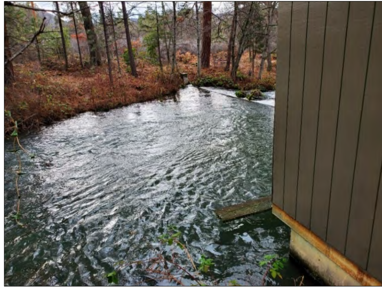
Figure 3-4. Intake Structure Location and City of Yreka Intake (Source: McMillen Jacobs)
