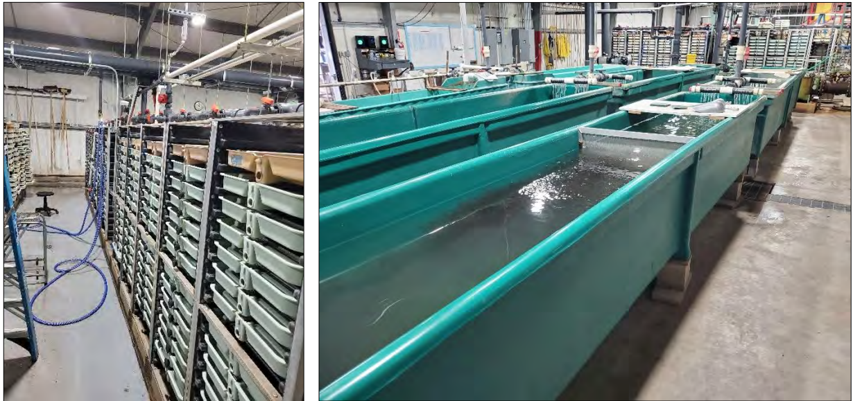
Figure 3-3. Existing IGFH Incubators (Left) and Working Vessels (Right) (Source: McMillen Jacobs)
