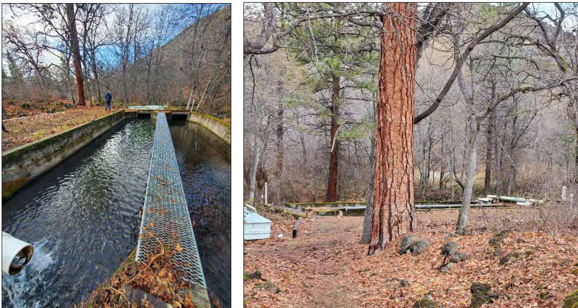
Figure 3-7. Existing Upper Raceway Bank (Source: McMillen Jacobs)
