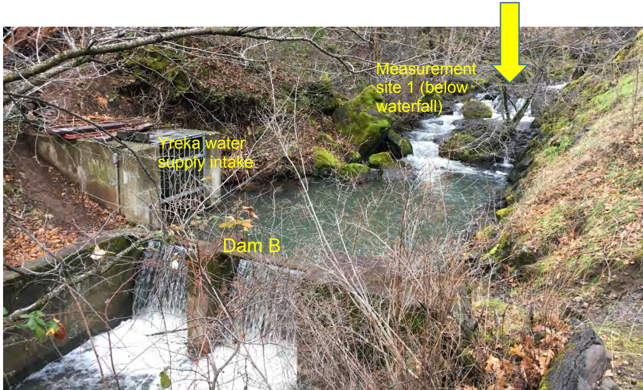
Picture 2: Dam B (upstream of Dam A)
