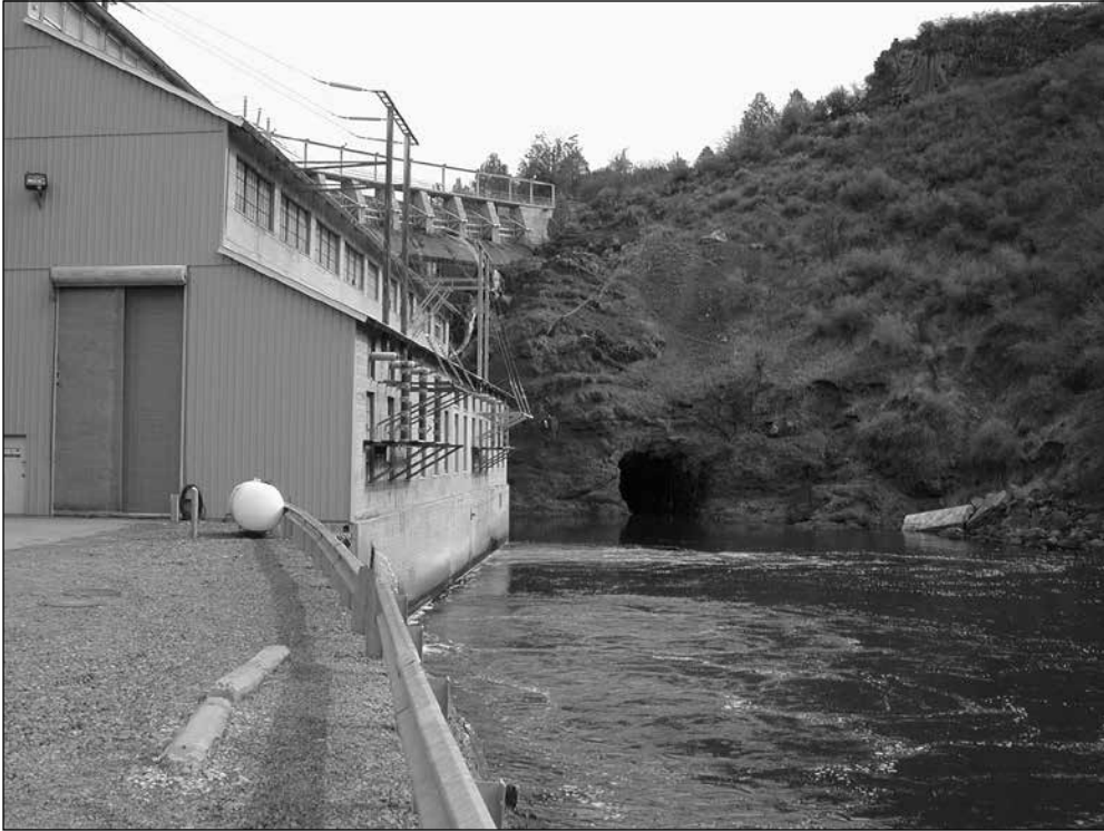
THE TUNNEL used to divert the Klamath River during the construction of Copco 1 Dam is still apparent. This photo was taken in 2003.
