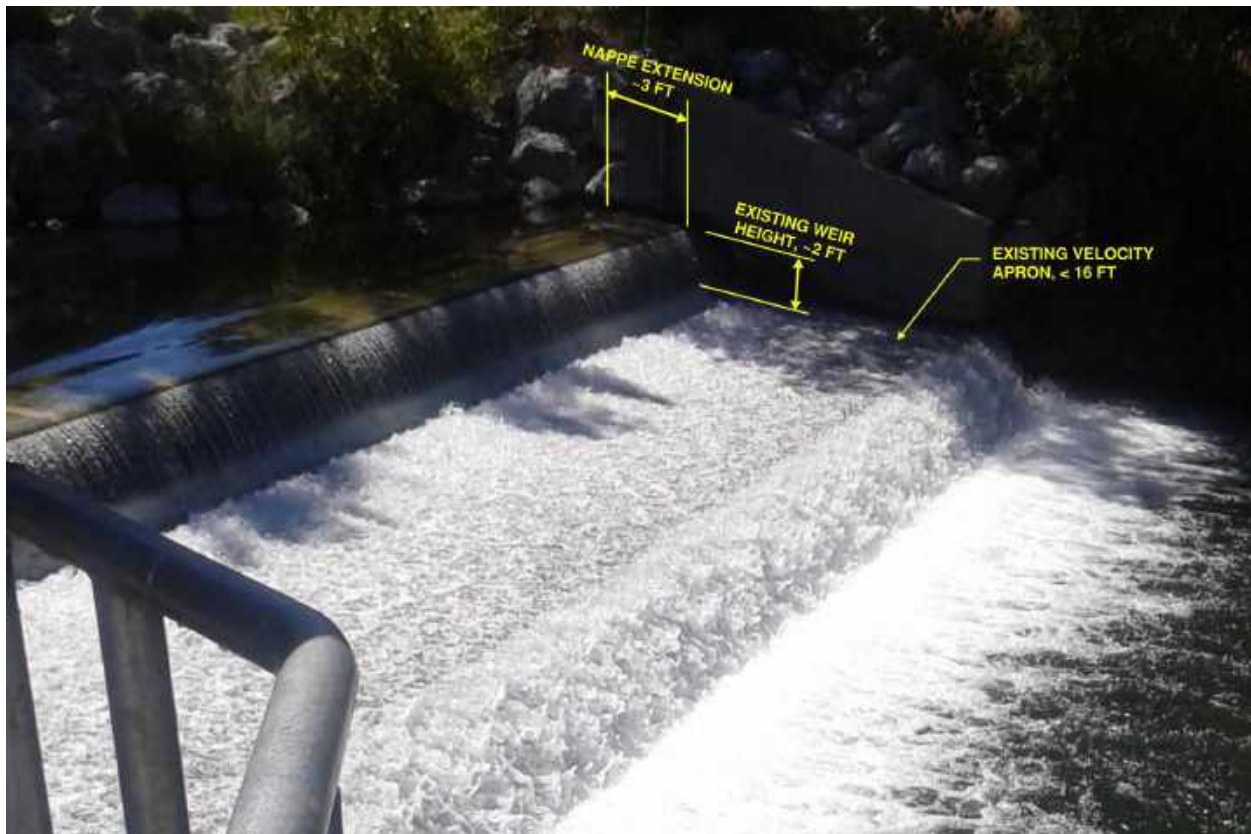
Figure 3-8. Nappe Extension Retrofit (Source; McMillen Jacobs)
