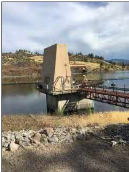
Photograph 5-3: Penstock Intake, Iron Gate
