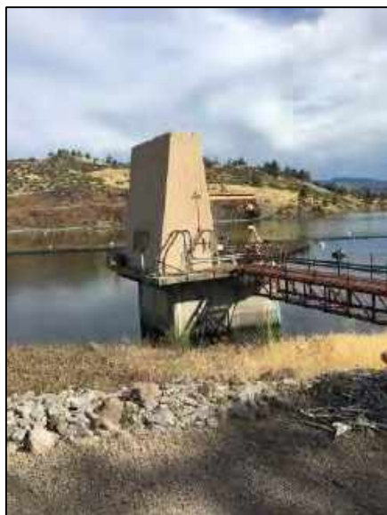
Photograph 5-3: Penstock Intake, Iron Gate
