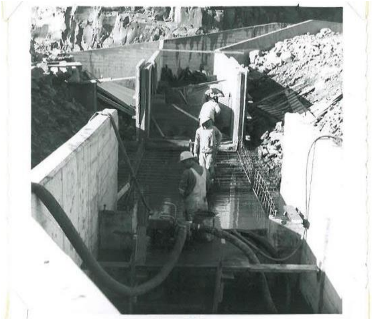
Figure 3-20 Iron Gate dam fish facilities, fish ladder construction, December 27, 1961 (PacifiCorp archive image IG-231)
