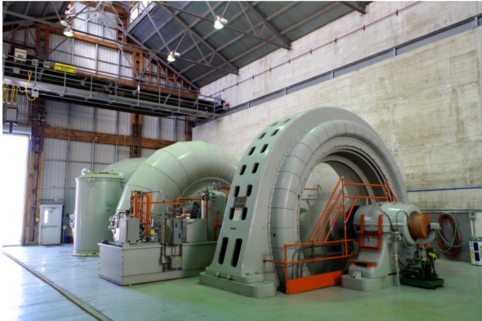
Photograph 3. Powerhouse interior, showing General Electric Generator Unit 2 and Allis-Chalmers turbines; view facing west, 2018.
