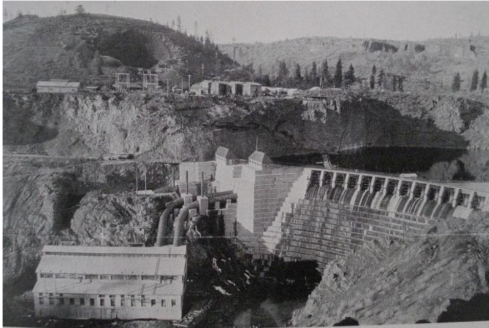
Photograph 15. Copco No. 1 in 1926, after the powerhouse was expanded, the dam was raised, Gatehouse No. 1 was rebuilt, Gatehouse No. 2 was built, and the single penstock was installed (Copco 1926b).
