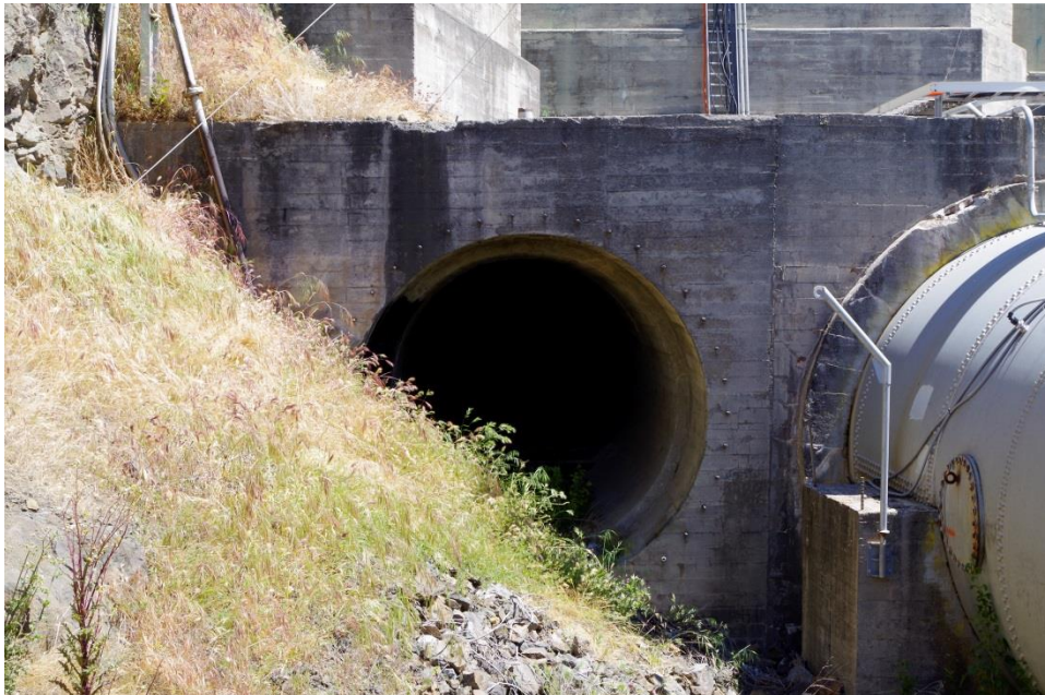
Photograph 4. Penstock section adjacent to the single penstock. This section would have accommodated an additional penstock to supply flow to a third generating unit. The additional penstock and third generating unit were never installed, 2018.
