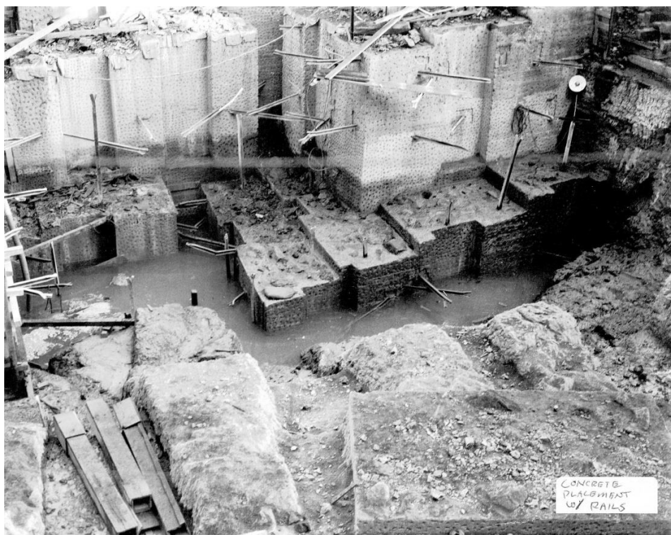
Photograph 9. Copco No. 1 Dam, showing the interlocking concrete block construction method, c.1916 (PacifiCorp archives image).
