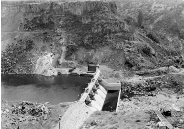
Figure 3-16 Copco No. 2 dam, showing original head gate and intake, undated photograph (courtesy of the Los Angeles Public Library, image LAPL00009700)
