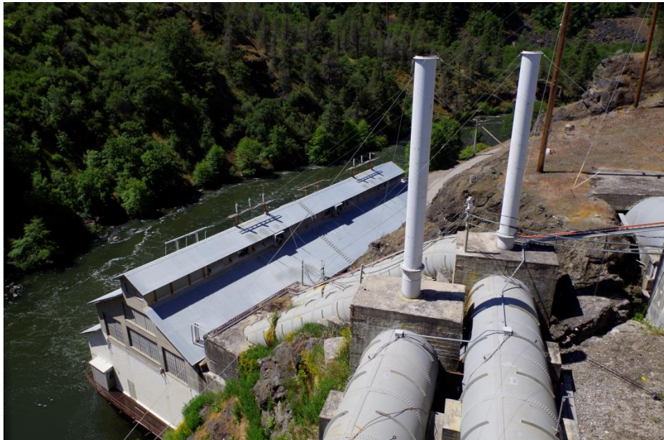
Photograph 2. Double penstock entering powerhouse, with single penstock at right; view facing southwest, 2018.
