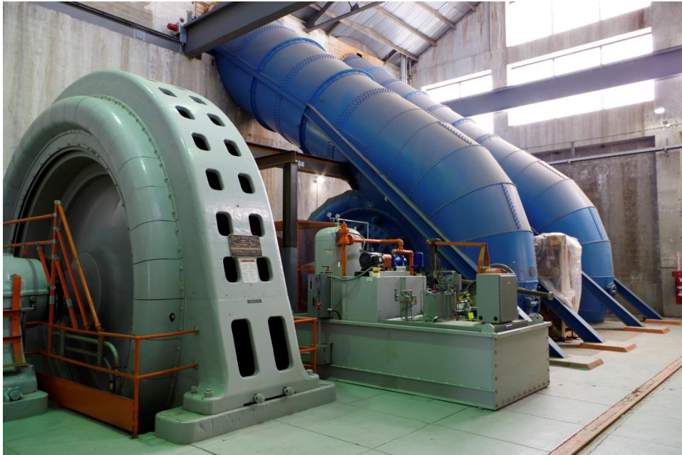
Photograph 5. Powerhouse interior, showing Generating Unit No. 1 and double penstock; view facing north, 2018.
