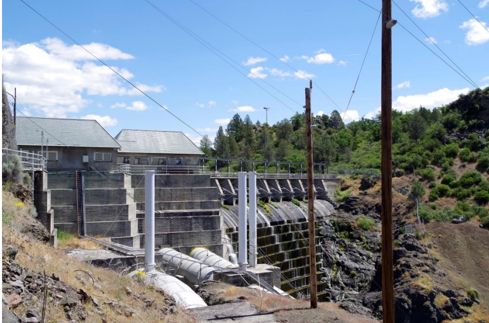
Photograph 3. Copco No. 1 dam, showing Gatehouse Nos. 1 and 2, single penstock, and double penstock; view facing east, 2018.
