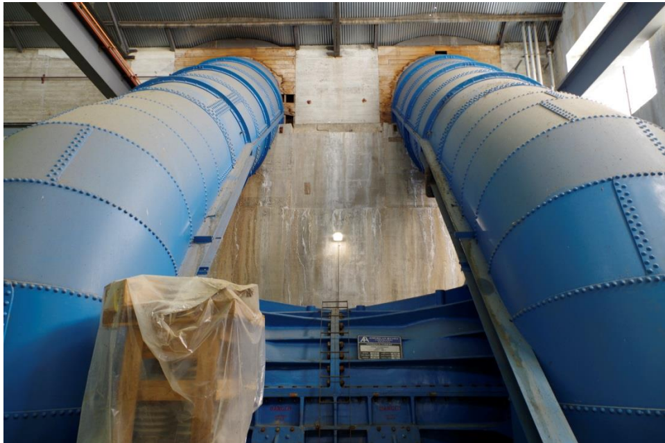
Photograph 4. Double penstock entering powerhouse interior; view facing northwest, 2018.
