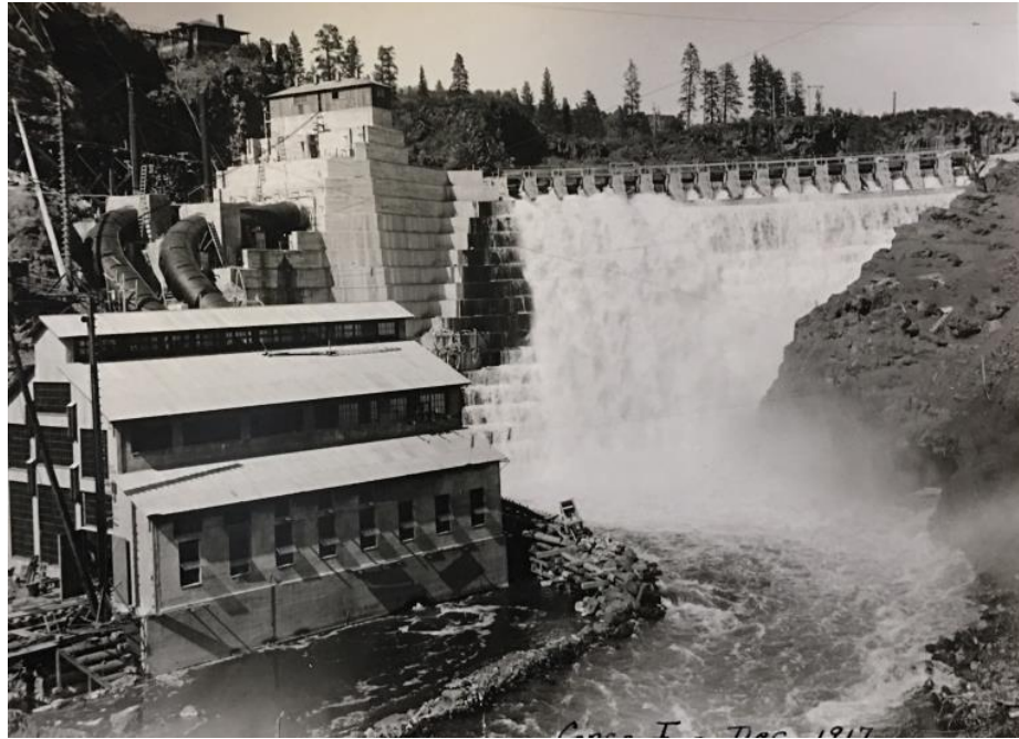
Photograph 11. The original appearance of the powerhouse, dam, and Gatehouse No. 1 in 1917, before the 1922 Copco No. 1 expansion (SOHS 1917). Note that dam had not yet been raised, Gatehouse No. 1 had not yet been rebuilt, Gatehouse No. 2 had not yet been built, and the powerhouse still had only eight windows on its river-facing elevation.
