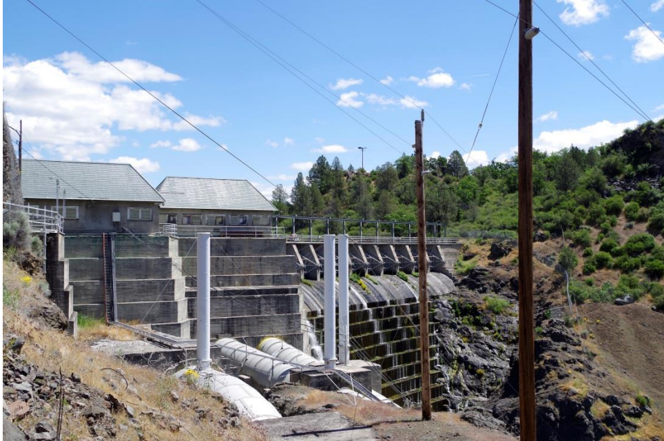
Photograph 1. Single penstock (foreground) and double penstock; view facing east, 2018.
