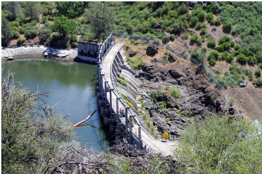
Photograph 2. Copco No. 1 Dam, showing gate hoist system along crest and diversion intake; view facing southeast, 2018.
