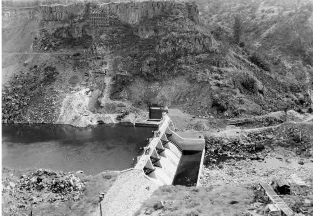
Photograph 11. Copco No. 2 Dam, showing original headgate and intake (LAPL n.d.). Timber cribbing visible on hillside.
