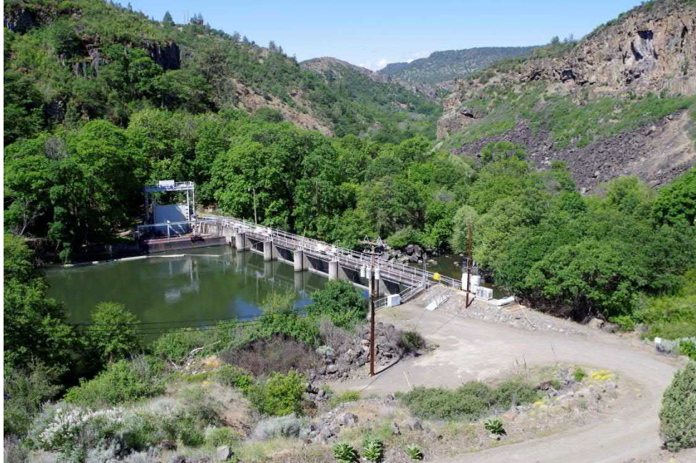
Photograph 1. Copco No. 2 Dam, showing head gate and intake at left; view facing downstream, 2018.
