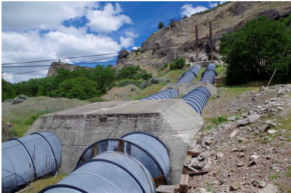
Photograph 4. Point where the water conveyance system transitions from the concrete tunnel to the double steel penstock; view facing northeast from powerhouse towards tunnel outlet in hillside, 2018.
