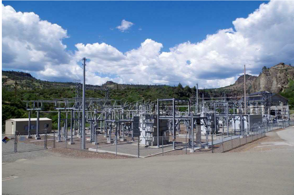
Photograph 5. Copco No. 2 Substation, showing control house at left, large transformers in center, and powerhouse in right background; view facing north, 2018. The substation was rebuilt in the early 2000s.
