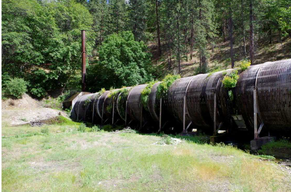
Photograph 12. Wood stave pipe, eastern end; view facing southeast, 2018.
