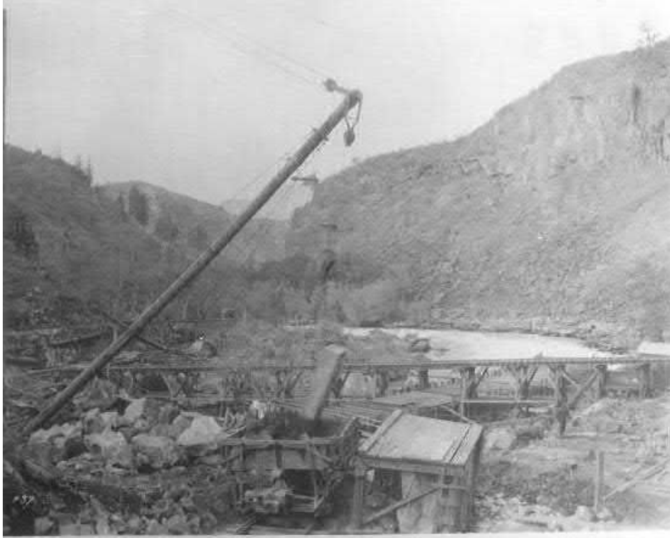
Photograph 9. Dumping of rock from dam excavation, 1924 (PacifiCorp archive image CO2-35).
