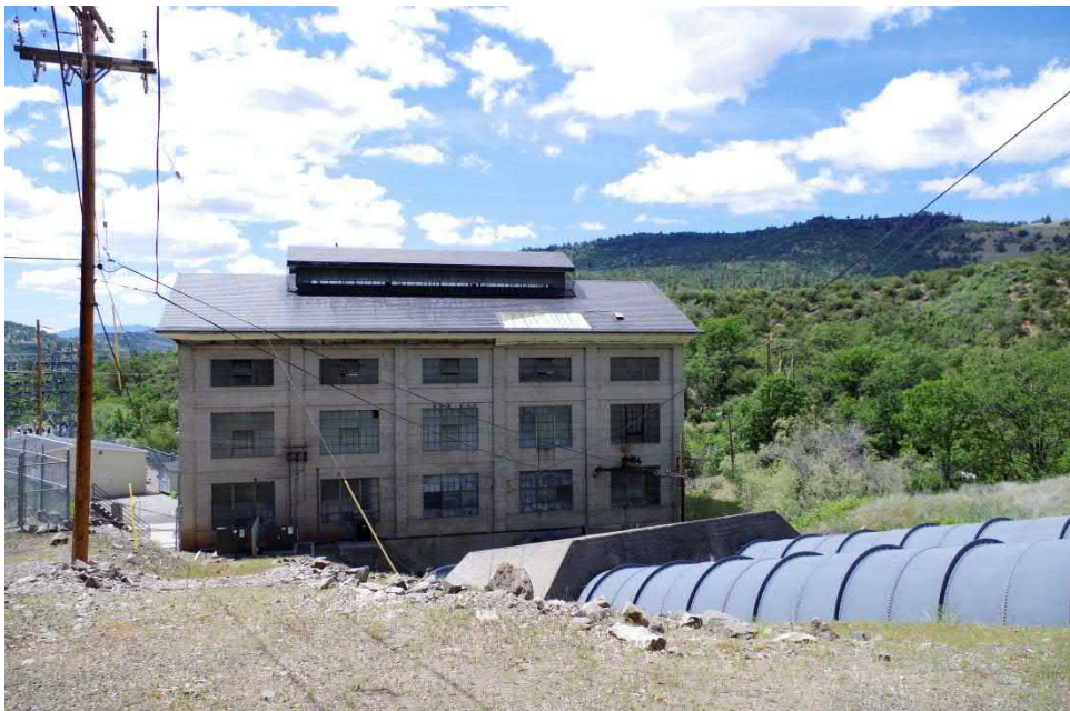
Photograph 4. Powerhouse, eastern elevation, showing control center (left) and penstock (right); view facing west, 2018.
