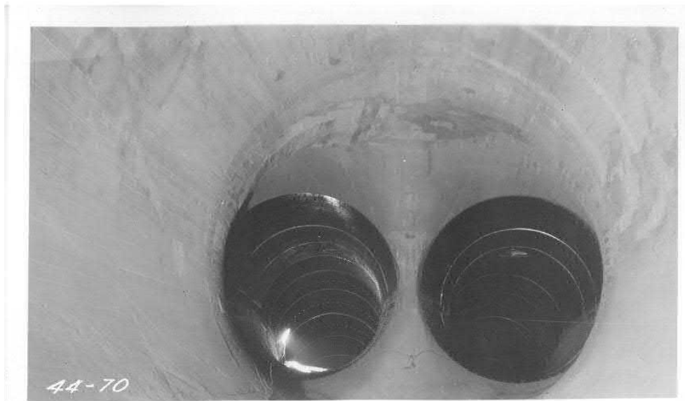
Photograph 10. Interior view of transition from concrete tunnel to double-steel penstock, July 18, 1925 (PacifiCorp archive image CO2-93).
