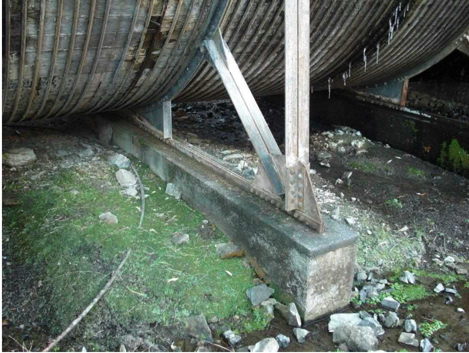
Photograph 14. Wood stave pipe, showing detail of concrete footing, 2018.
