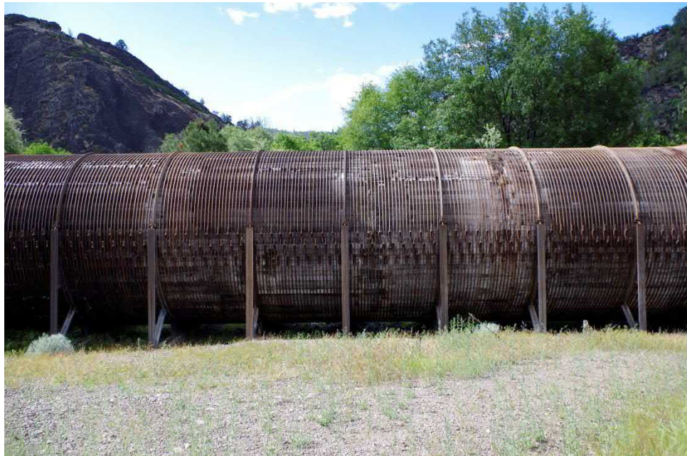
Photograph 13. Wood stave pipe, western end; view facing northwest, 2018.
