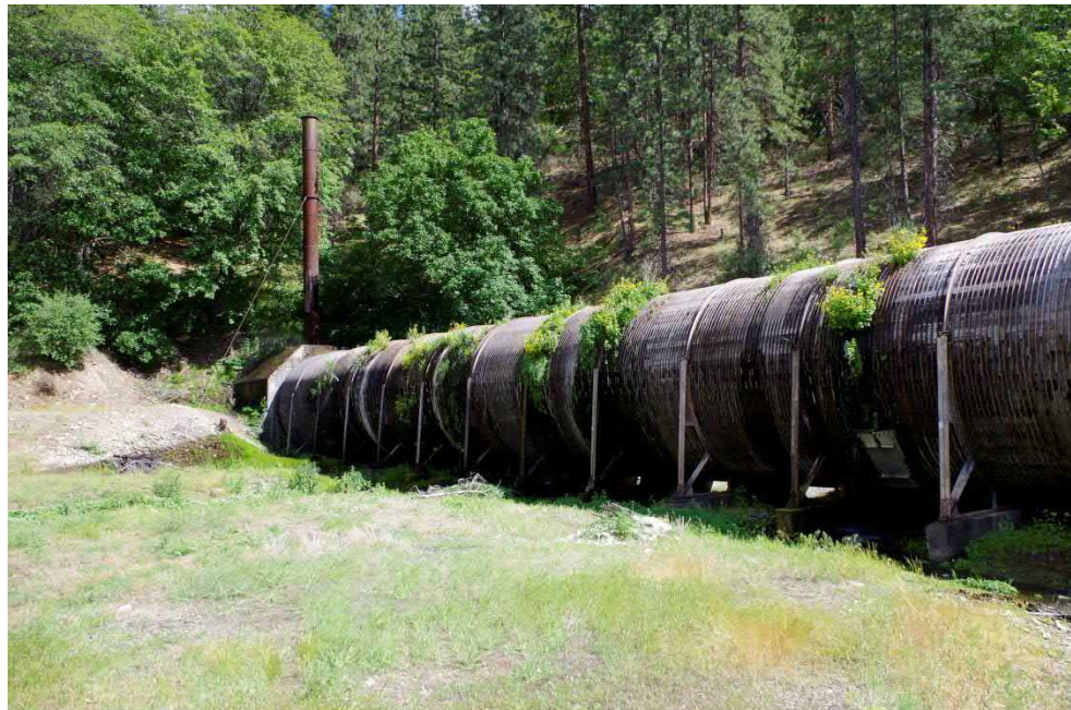
Photograph 2. The eastern end of the wood-stave pipe, where the water conveyance system transitions from the concrete-lined tunnel to the wood stave pipe; view facing southeast, 2018.
