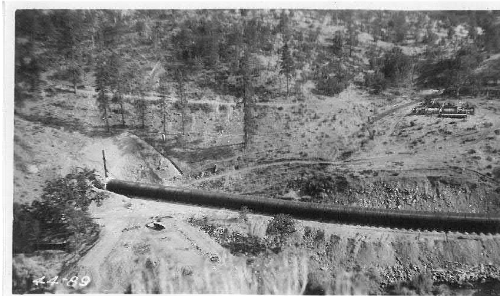
Photograph 9. Eastern half of the completed wood stave pipe, showing what appears to be a construction camp in right background, August 1, 1925 (PacifiCorp archive image CO2-95). At left, the wood stave pipe transitions to the concrete tunnel.
