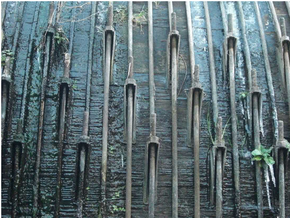
Photograph 15. Wood stave pipe, detail of wood staves and steel bands, 2018.
