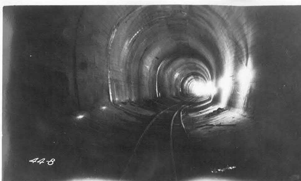
Photograph 8. Concrete-lined tunnel, June 15, 1925 (PacifiCorp archive image CO2-84). The intake supplies flow to the subterranean concrete-lined tunnel. The concrete tunnel emerges and transitions to wood stave pipe.
