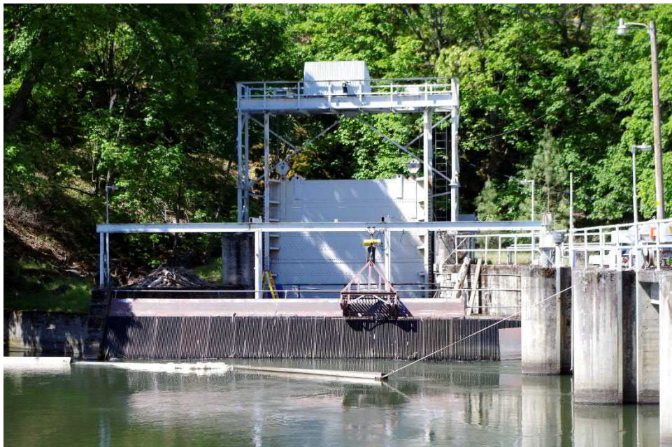
Photograph 2. Copco No. 2 Dam, showing the 1996 headgate and tunnel intake; view facing southwest, 2018.
