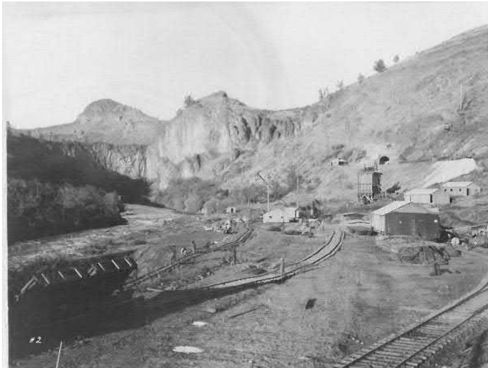
Photograph 10. Construction at Powerhouse site, showing Klamath River, Lower Camp/Camp 2, Klamath Lake Railroad spur, tall rock-crushing plant, and concrete tunnel outlet (PacifiCorp archive image CO2-19).
