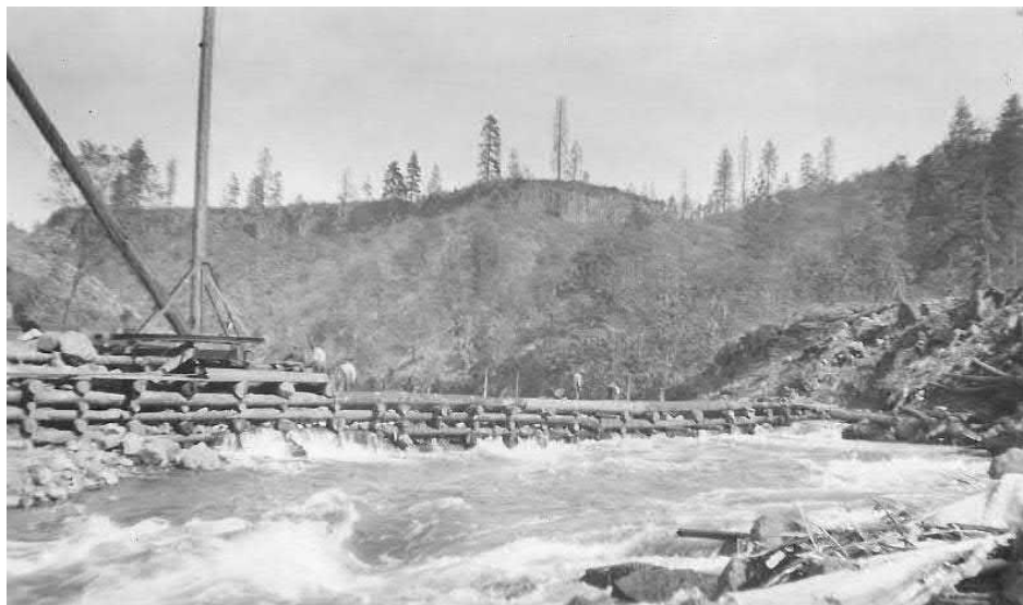
Photograph 12. Coffer dam used during construction, September 6, 1924 (PacifiCorp Archive image CO2-78).
