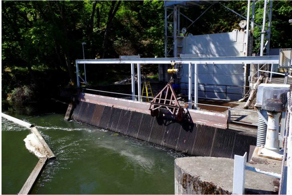
Photograph 1. The water conveyance system begins at the intake for the concrete-lined tunnel at the Copco No. 2 Dam. This 2018 image shows the intake, with head gate in background; view facing south. Water that flows through the intake flows from the small, unnamed reservoir extending 0.3 mile between the Copco No. 1 and Copco No. 2 Dams.
