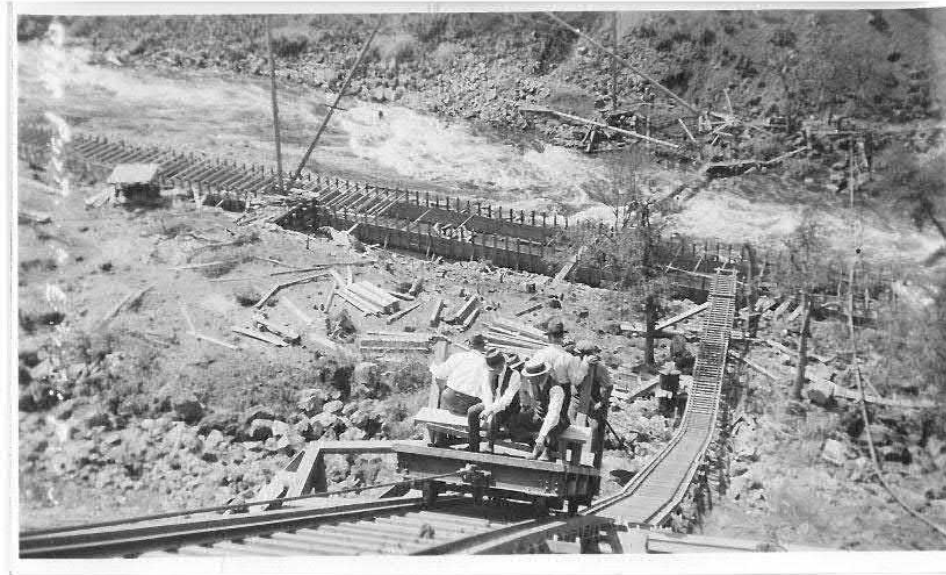
Photograph 19. Tramway for delivery of construction materials to Copco No. 2 Dam site, showing Paul McKee (Copco chief executive officer) and Mr. Kemmach, August 15, 1924 (PacifiCorp archive image CO2-111).
