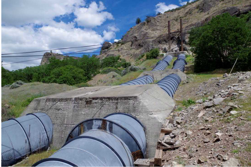
Photograph 3. The water conveyance system transitions from the concrete tunnel to the double steel penstock; view facing northeast from powerhouse towards tunnel outlet in hillside, 2018.
