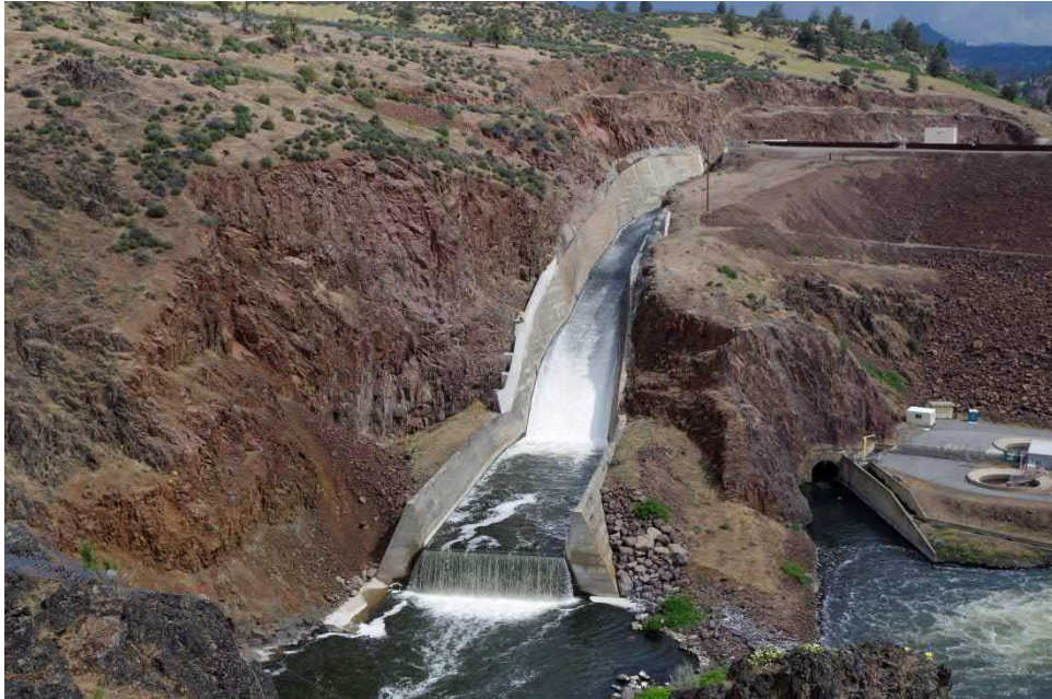
Photograph 5. Spillway chute; view facing northeast, 2018. Diversion tunnel visible at lower right.
