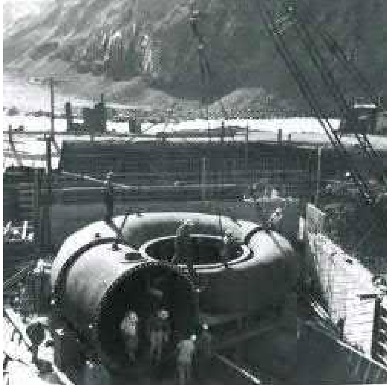
Photograph 9. Powerhouse scrollcase installation, August 22, 1961 (PacifiCorp archive image IG-141).
