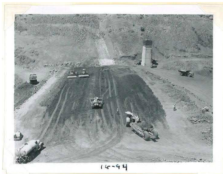
Photograph 8. Rolling clay on the dam, July 25, 1961 (PacifiCorp archive image IG-94).
