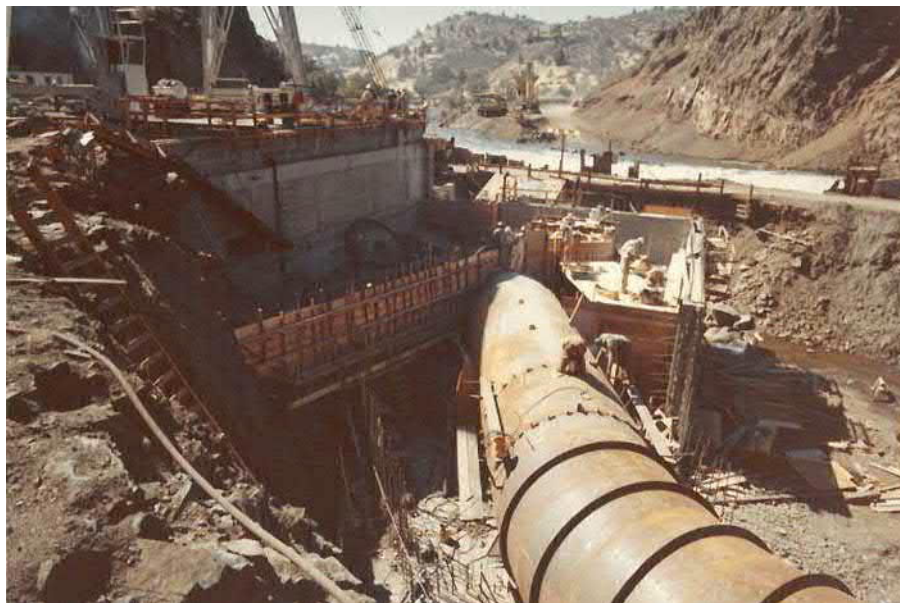
Photograph 6. Penstock where it enters powerhouse, September 1961 (PacifiCorp archive image IG-167).
