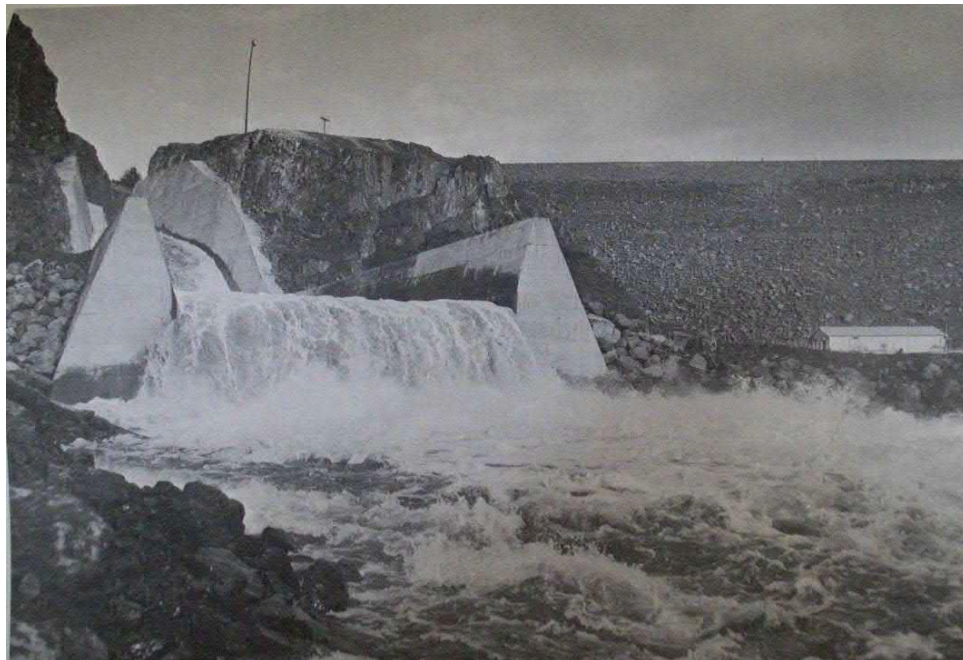
Photograph 12. Spillway chute outlet in 1965 after destructive December 1964 flooding repairs (Pacific Power 1965:5407-R19).
