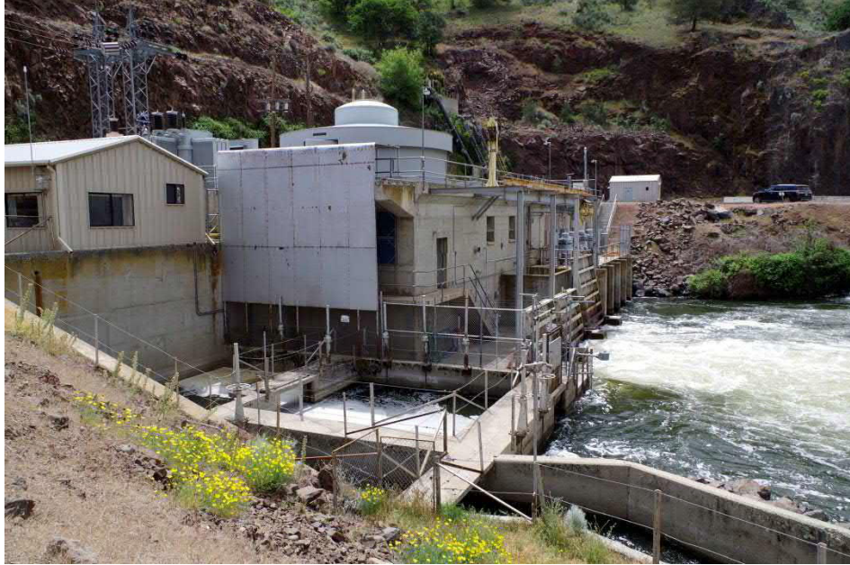
Photograph 3. Powerhouse, showing fish ladder in foreground, communications building at left, and generator deck; view facing southeast, 2018. The fish collection area is visible in the foreground at the entrance to the fish ladder.
