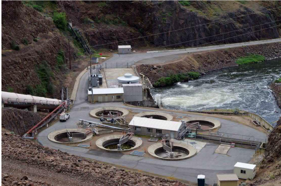
Photograph 1. Dam fish facilities, from left showing water supply pipe adjacent to penstock and spawning building surrounded by six holding ponds; view facing south, 2018. The aerator is visible in the left background along the hillside. Pond #1 is in the right foreground. Pond #6 is in the left background (Logan and Hankin 2008:9).
