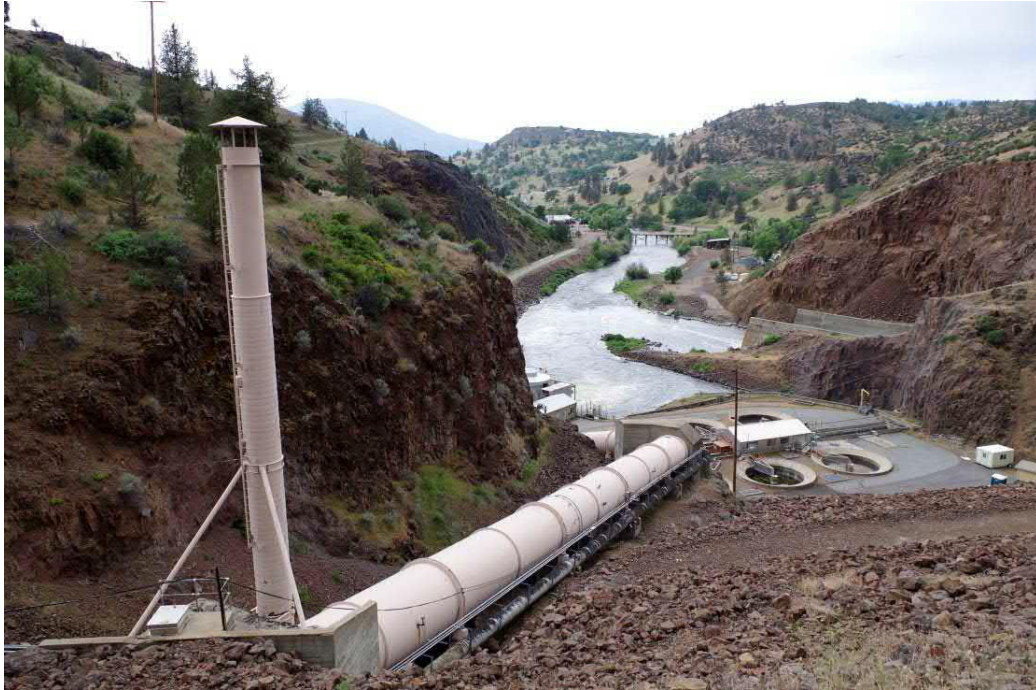
Photograph 3. Penstock; view facing southwest from the dam crest, 2018. The spawning building is surrounded by the six holding ponds, and the Klamath River is visible in the background.
