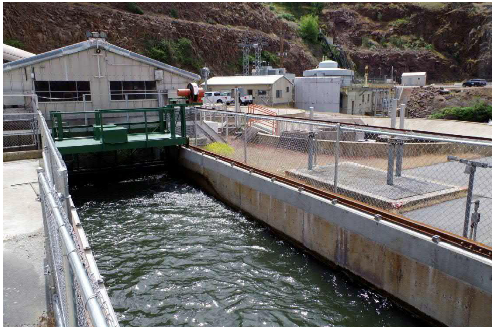
Photograph 4. Fish trap, where fish arrive after ascending the fish ladder and remain before they are moved into the spawning building; view facing southeast, 2018.
