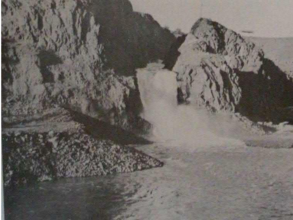
Photograph 11. Spillway chute outlet in January 1962 (Pacific Power 1962a).
