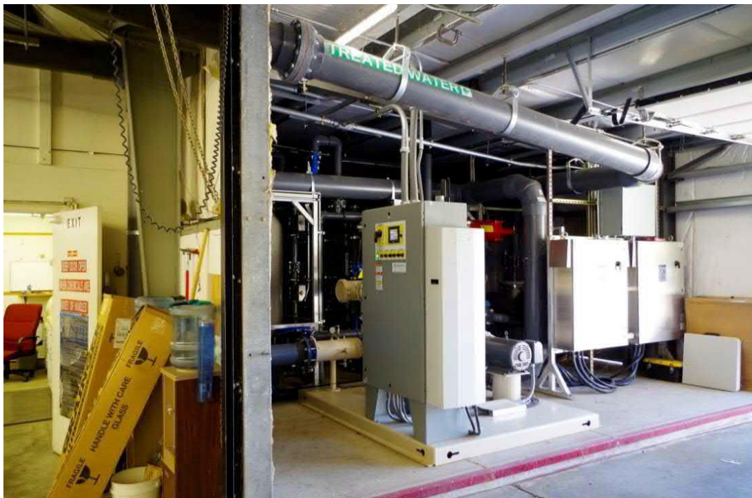
Photograph 6. Hatchery building 2015 addition interior, showing water filtration system; view facing south, 2018.
