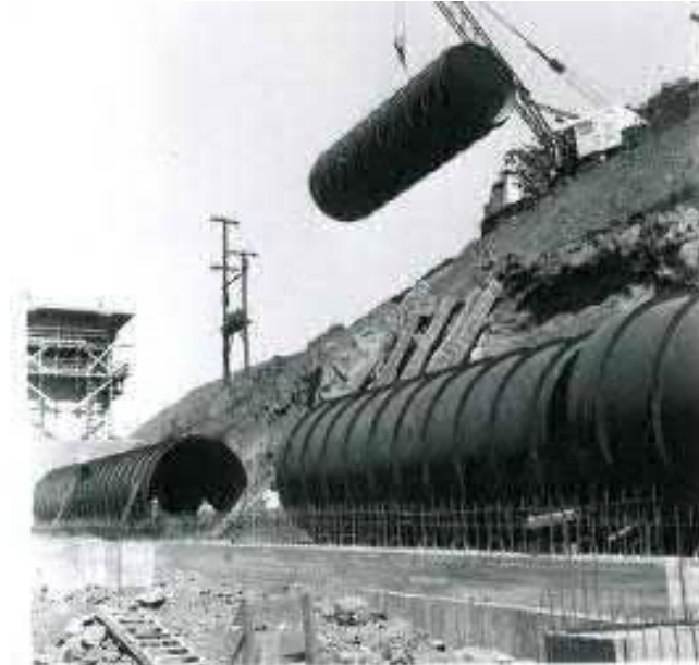
Photograph 9. American Pipe and Construction Company assembling penstock pipe for embedded sections, July 20, 1961 (PacifiCorp archive image IG-131).
