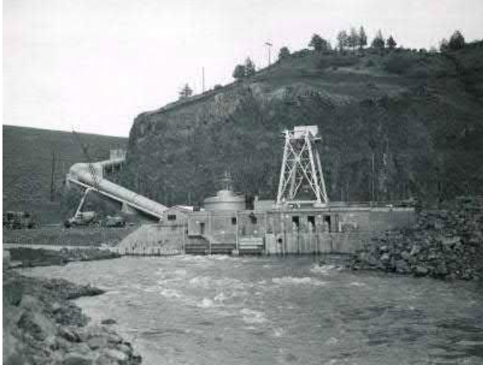
Photograph 7. Powerhouse, showing penstock at left; view facing northeast, January 1962 (PacifiCorp archive image IG-243). The gantry crane is currently located at the J.C. Boyle Powerhouse in Southern Oregon.
