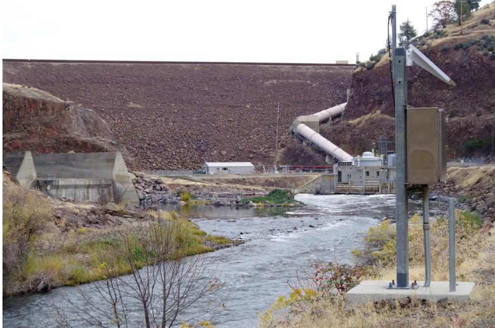
Photograph 1. Iron Gate Dam; view facing north, 2018. Concrete spillway channel outlet at left, spawning building in center, and penstock entering powerhouse at right.
