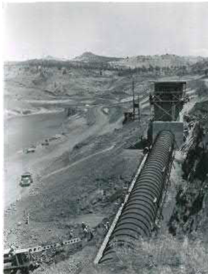
Photograph 10. Penstock and intake structure, July 25, 1961 (PacifiCorp archive image IG-117).
