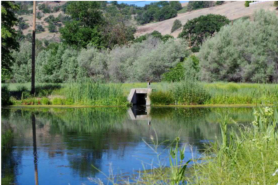
Photograph 20. Southernmost settling pond on the southern side of Bogus Creek, showing concrete bulkhead through which discharge drains into the Klamath River; view facing west. Transmission line wood pole visible at left, 2018.
