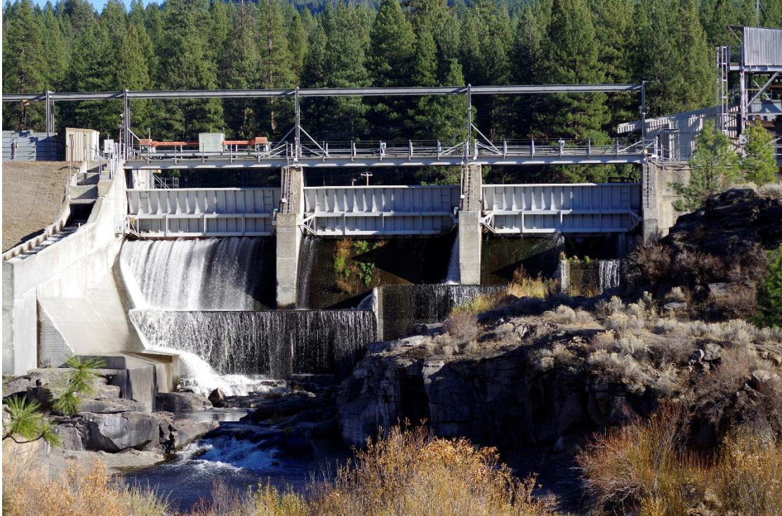
Photograph 7. Gated spillway and diversion culvert; facing east, 2018
