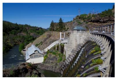
Figure 4-2 Copco No. 1, showing powerhouse, dam, and gatehouse no. 1
