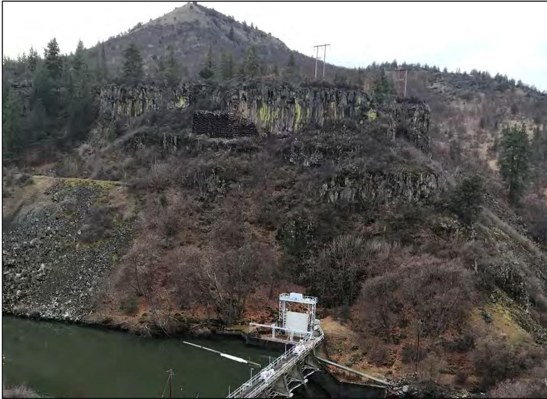
**Figure 4.8** Cliff Band and Timber Crib above Intake Structure
