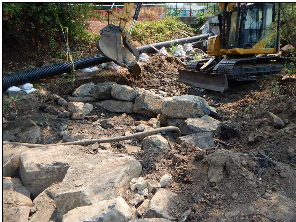
Photograph 1.5 Larson Creek Example of Boulder Buttress Construction
