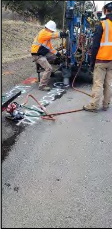
Photograph 11. Looking at asphalt coring at Road Core RC-CR-004 (STA 315+66.0).
