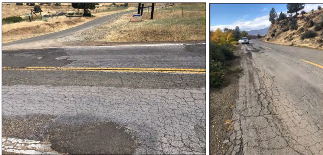
Figure 6.2 Copco Road Asphalt and Basecourse Replacement Repair Examples
