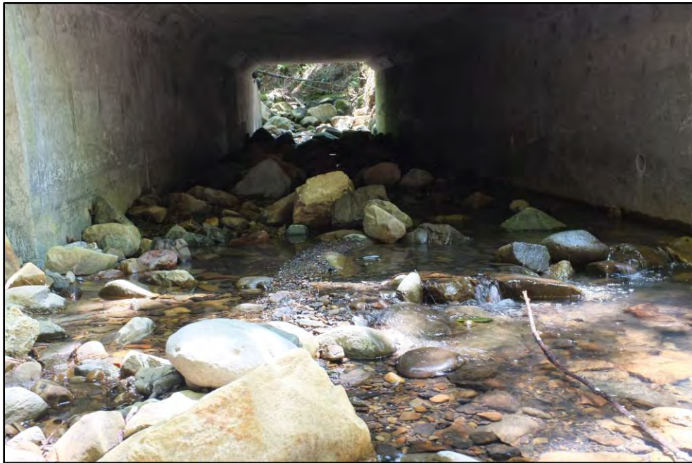
Photograph 1.4 Sunken Box Culvert with Engineered Streambed Material Example
