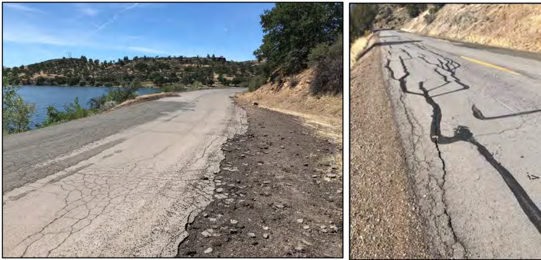
Figure 6.1 Copco Road Mill and Overlay Repair Examples
