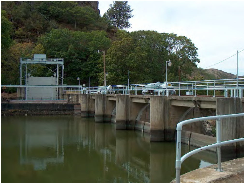
Fig. 1 Diversion Dam, Spillgates, and Intake Structure
