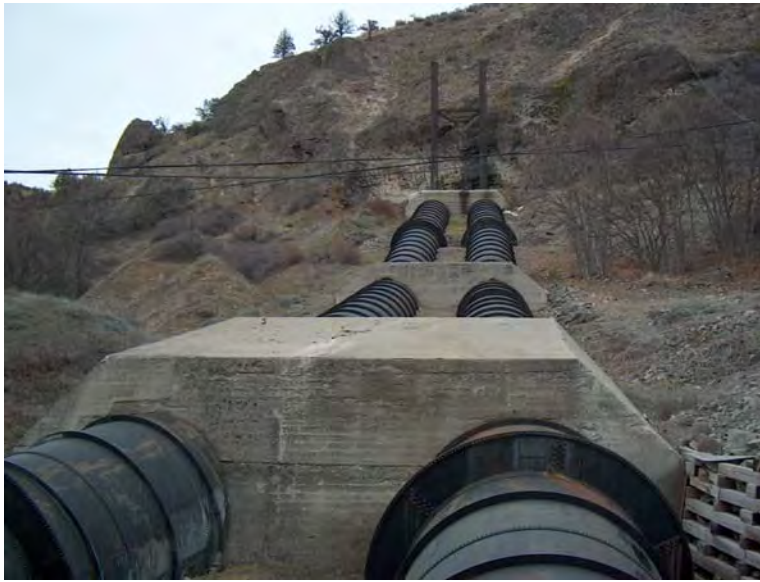
Fig. 3 Penstocks Exiting Tunnel
