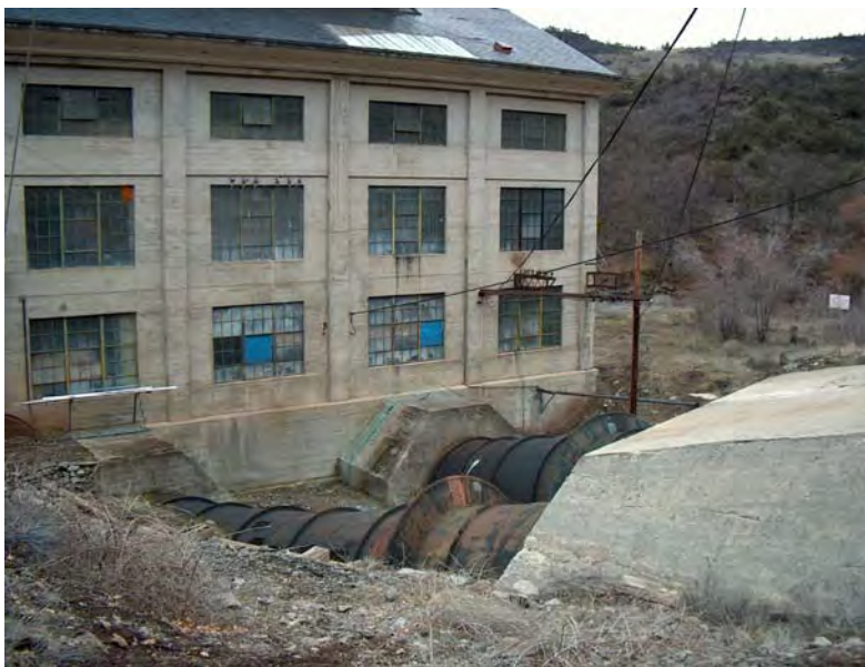
Fig. 4 Penstocks Entering Plant
