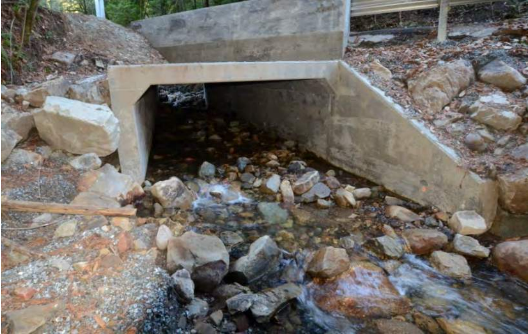
Image 4. Corrolitos Creek Sunken Box Culvert
