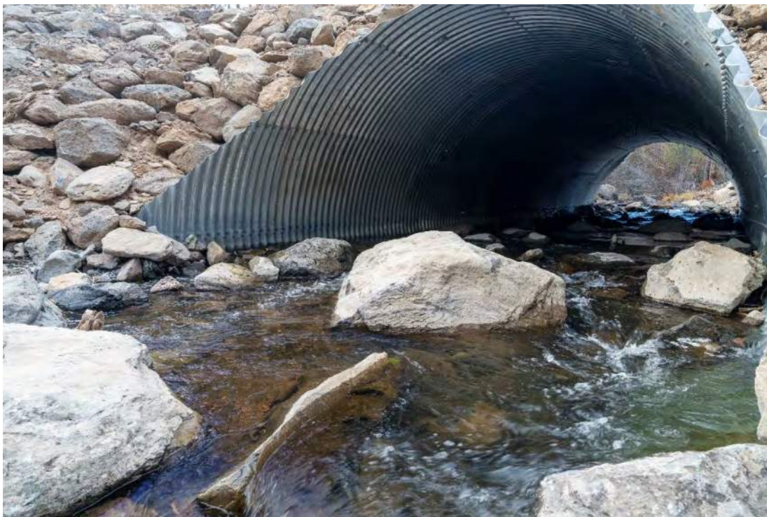
Image 3. Elder Creek Multi-plate sunken culvert (span 21 ft, rise 13 ft)
