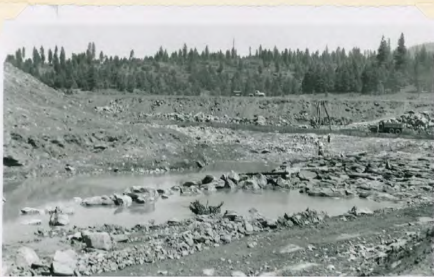
Dam. Unwatered foundation. 7/25/57
