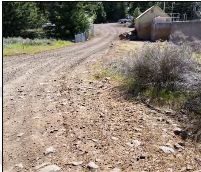
Figure 2.13 Evidence of little to no gravel surfacing along access roads. Coarse fraction in subgrade include cobble to boulder sized particles
