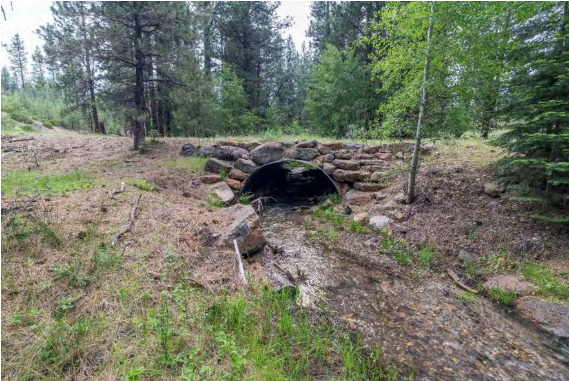
Image 5. Howard Creek Tributary sunken culvert (span 12 ft, 8 ft rise)
