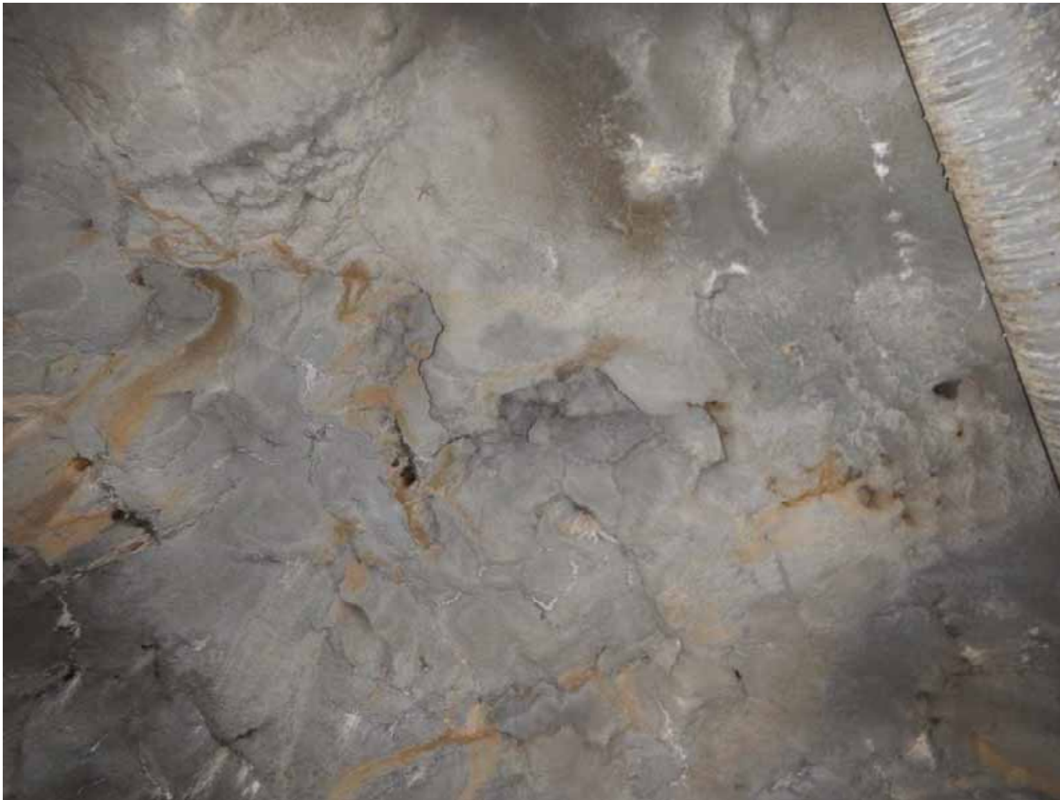
Profile of the tunnel crown in the shotcreted section is locally highly irregular suggesting the presence of a 'loose' closely jointed rock mass with previous crown instability
