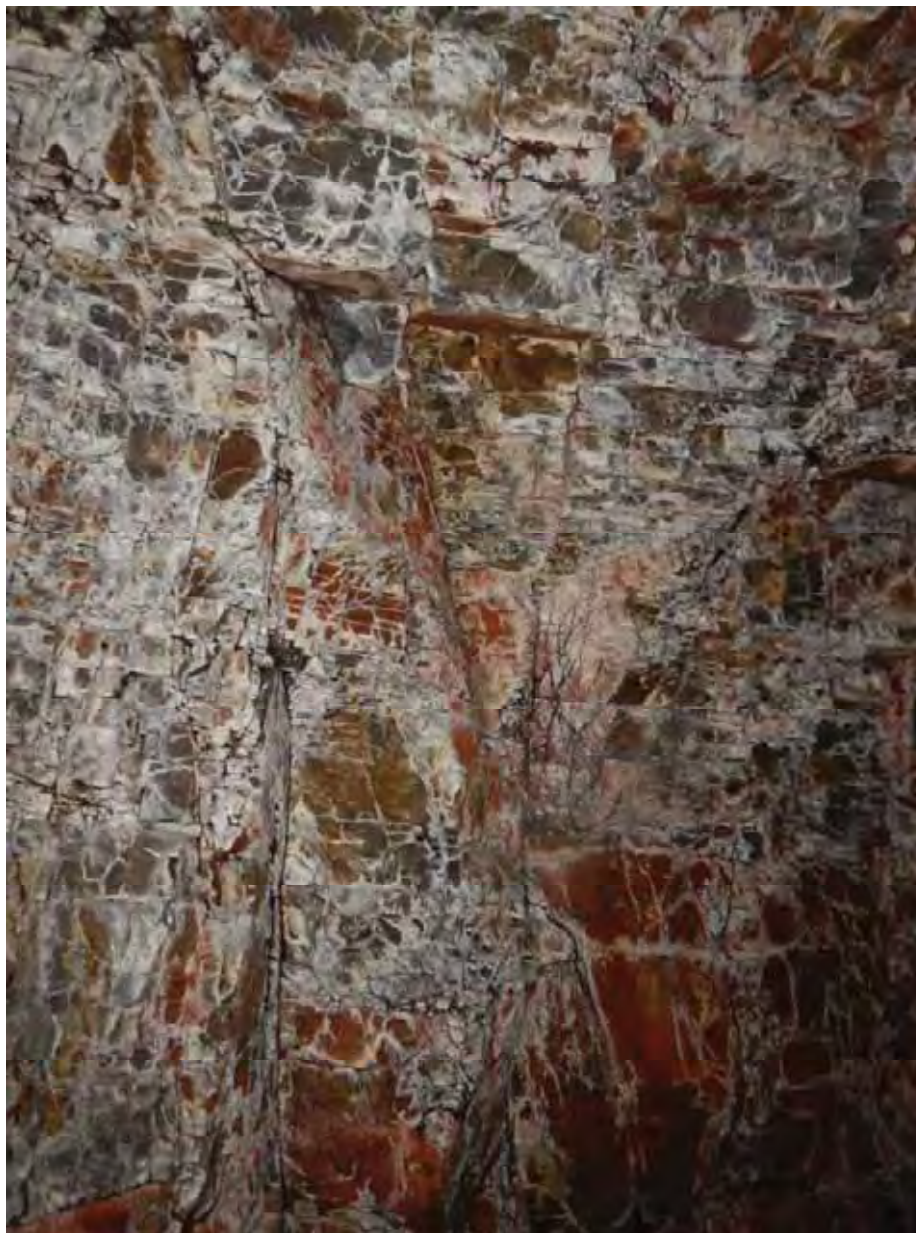
STA 380.6 ft - Triangular 53 ft 3 wedge failure at crown/wall interface in area with very closely to closely spaced joints. The wedge was formed by the intersection of low angle Set 3 Joint with steep joints
