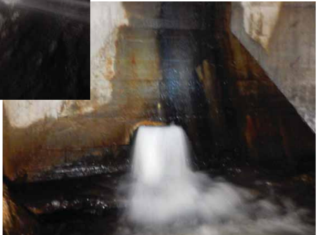
STA 176.5 ft - Tunnel Plug - Water flow at tunnel crown and from valve
