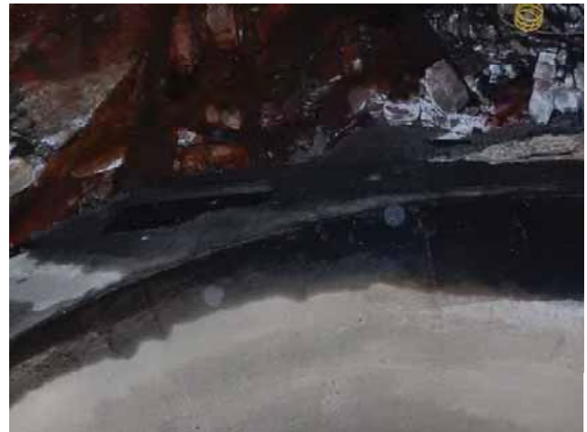
STA. 516.7 ft – Seepage observed around Upstream Concrete Liner
