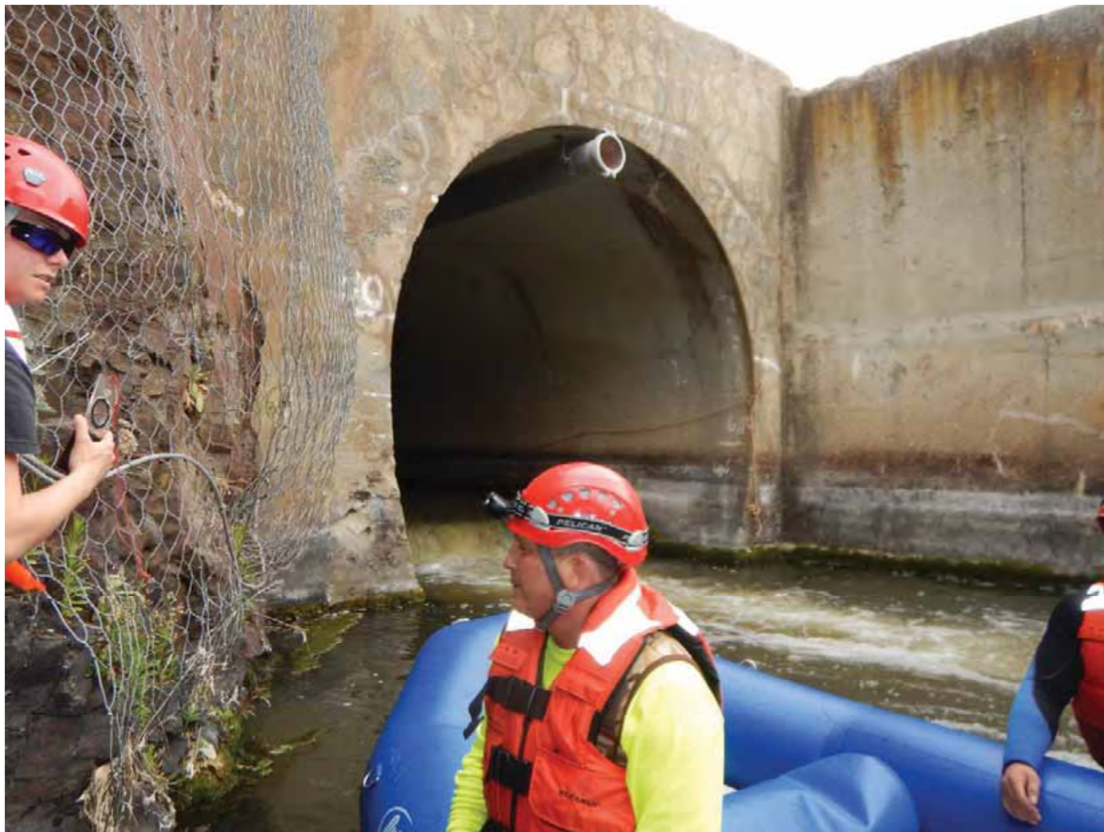
Concrete Lining and Ventilation Pipe at Downstream Portal
