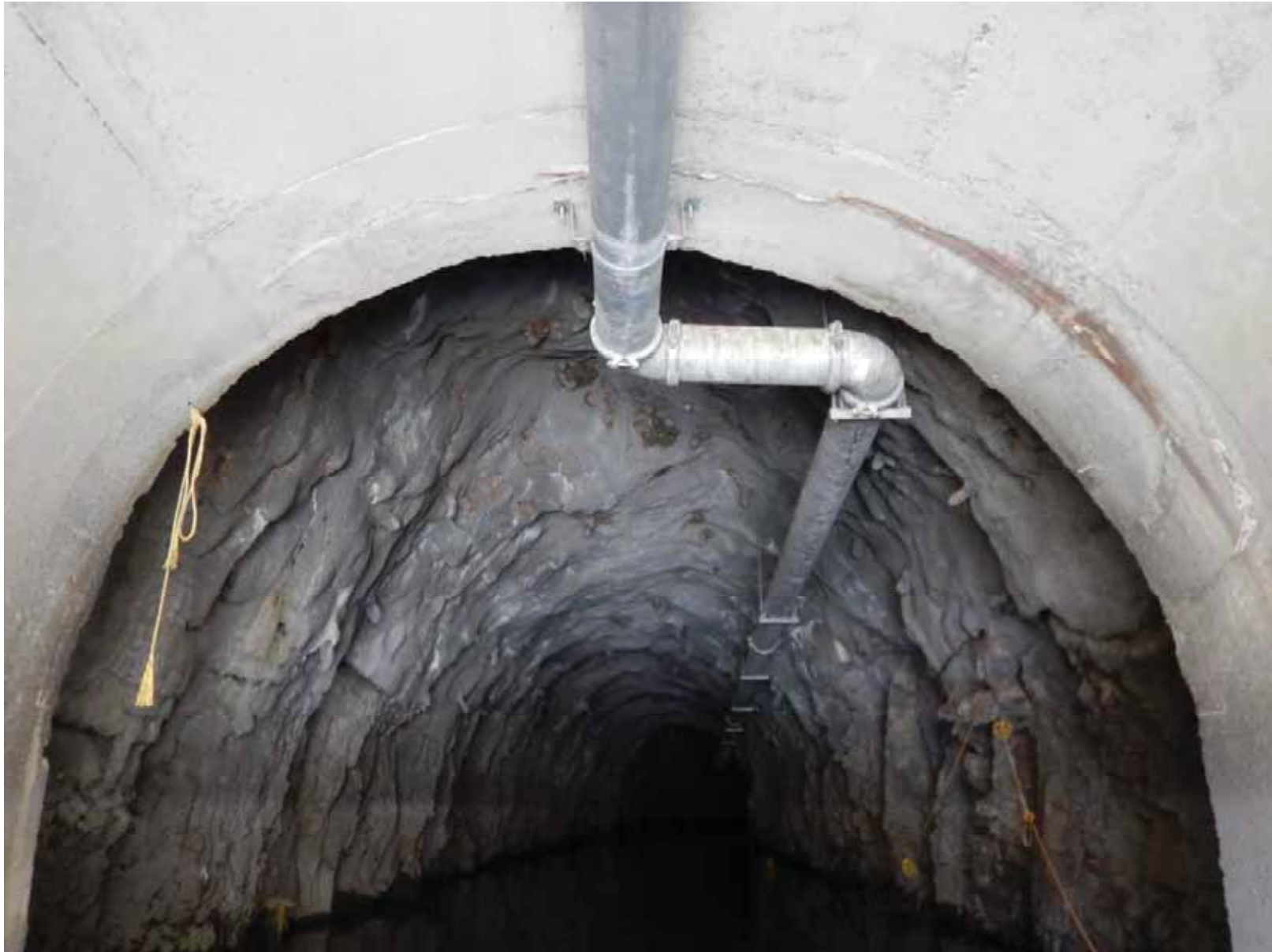
Downstream Concrete Liner and Ventilation Pipe
