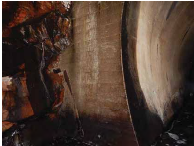
STA. 516.7 ft – Seepage observed around Upstream Concrete Liner
