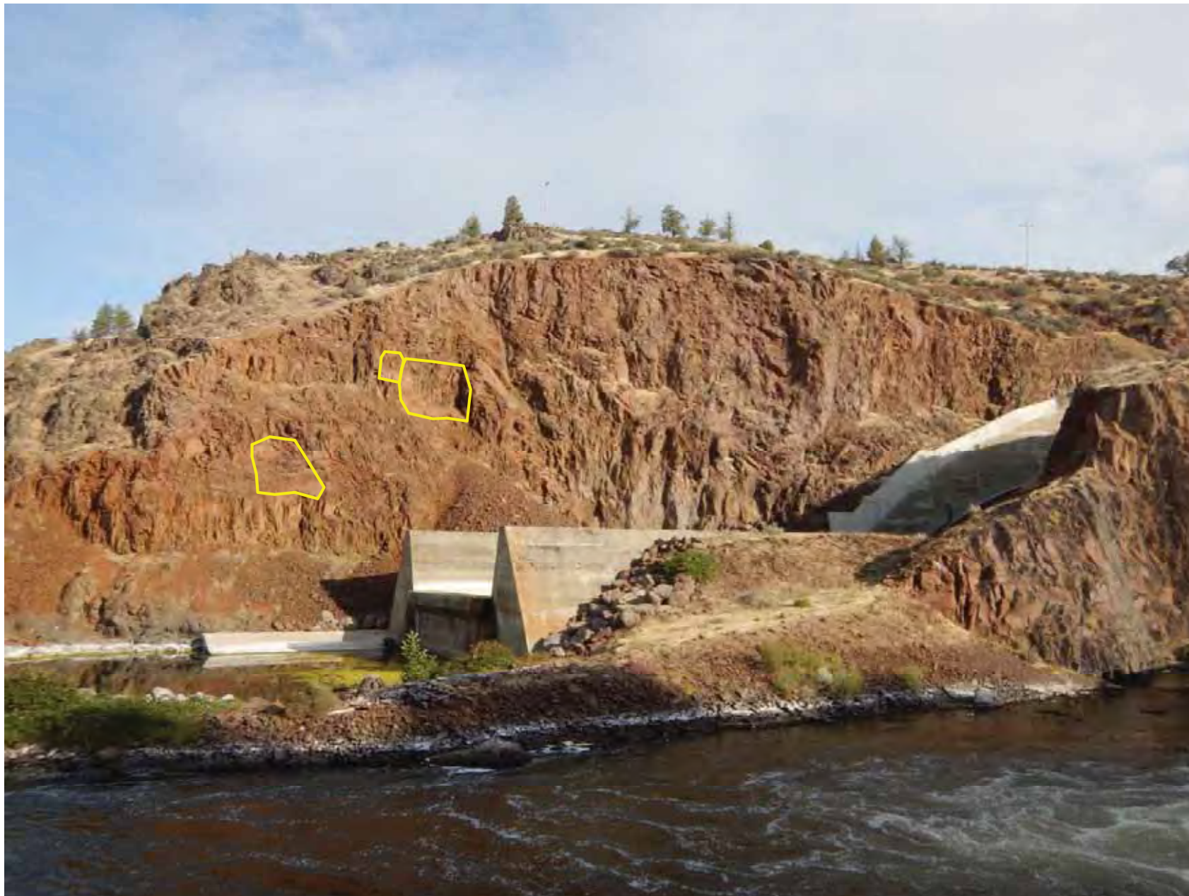
Rock Slides have occurred in the Rock Cut above the Spillway
