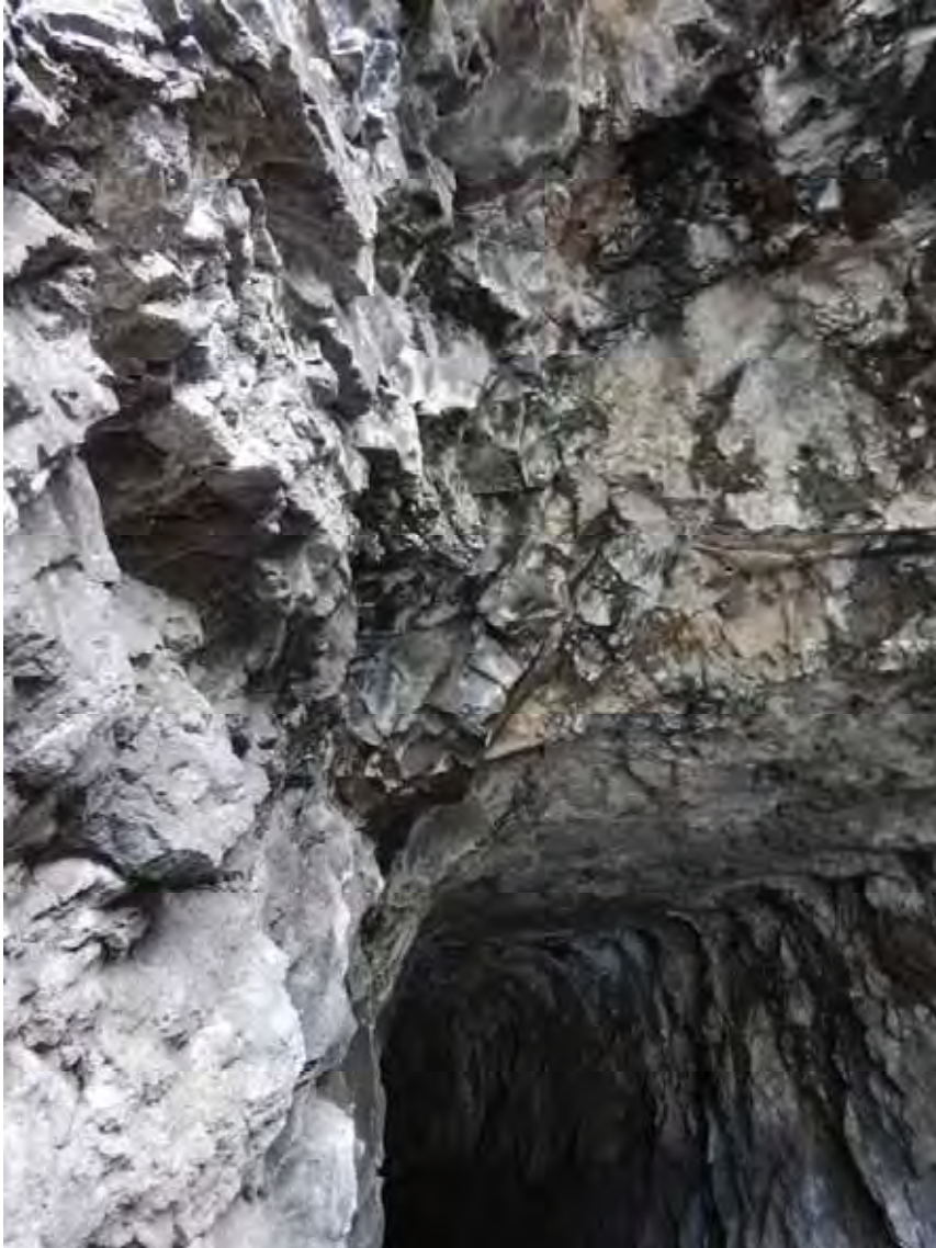
Overbreak observed in the first 15 ft of the Tunnel Crown from the Portal.
