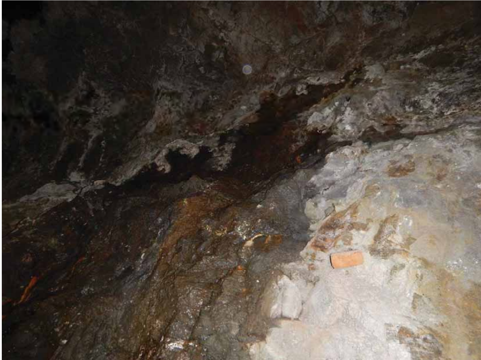
STA. 144.4 ft – Seepage from Set 1 Joint
