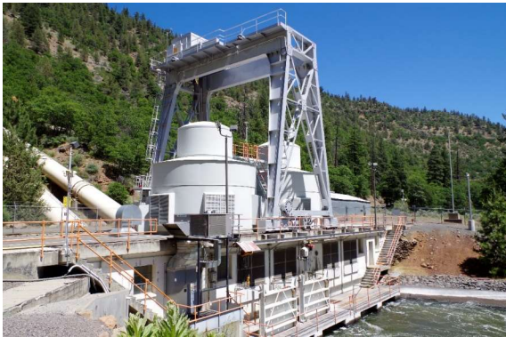
Figure 0-1 J.C. Boyle powerhouse
