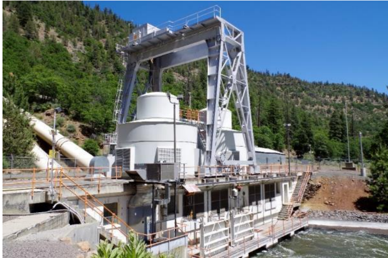
Figure4-1 J.C. Boyle powerhouse
