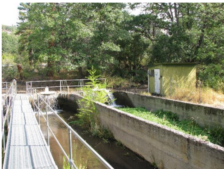
Figure 4-5 Fall Creek Hatchery, 1937 raceways and former incubation shed
