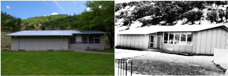
Figure 0-2 Fall Creek School, 2018 (left) and circa 1965 (right)
