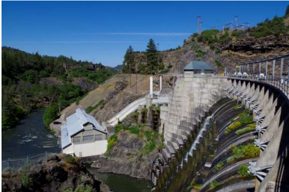
Figure 0-2 Copco No. 1, showing powerhouse, dam, and gatehouse no. 1
