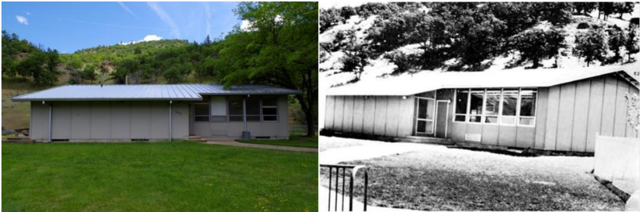
Figure 7-2 Fall Creek School, 2018 (left) and circa 1965 (right)
