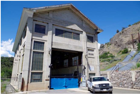
Figure 0-3 Copco No. 2, showing powerhouse and penstock
