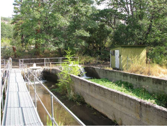
Figure 0-5 Fall Creek Hatchery, 1937 raceways and former incubation shed
