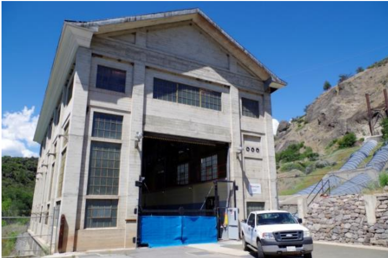
Figure 4-3 Copco No. 2, showing powerhouse and penstock
