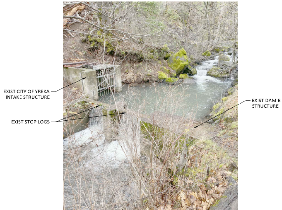
Figure 3. Dam "B" Intake Photograph
