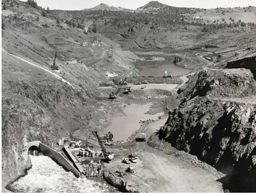
Figure D-10. View Looking Upstream at Site of Iron Gate Dam during Construction and Showing Reservoir Area
