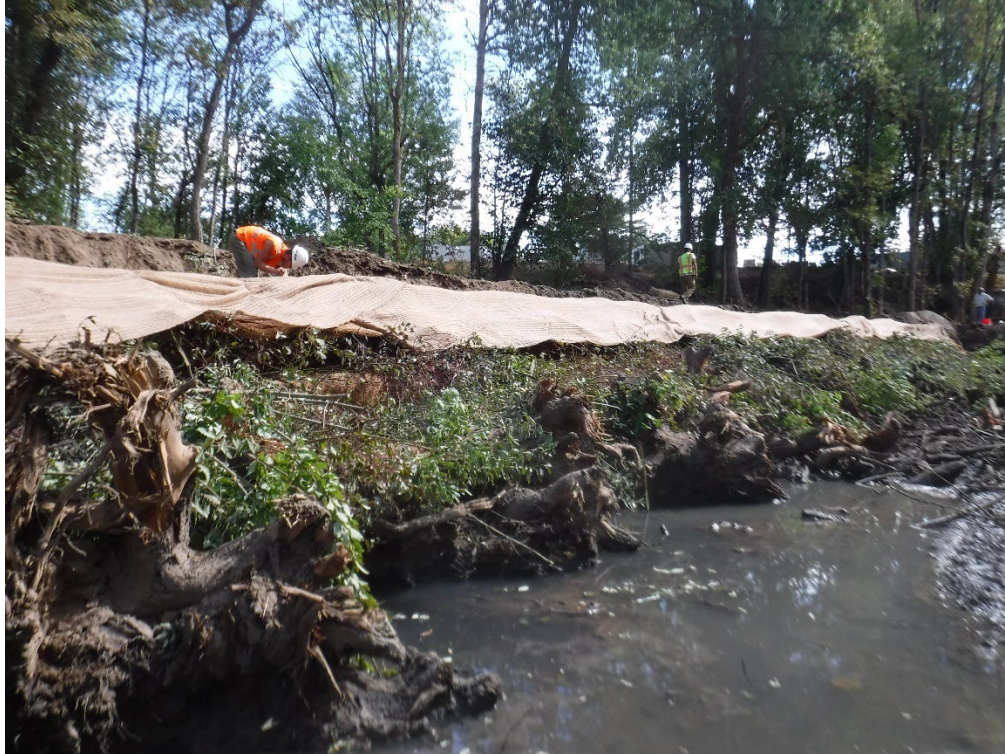
Figure 5-2. Example of Toe Wood Being Installed to Improve Fringe Complexity
