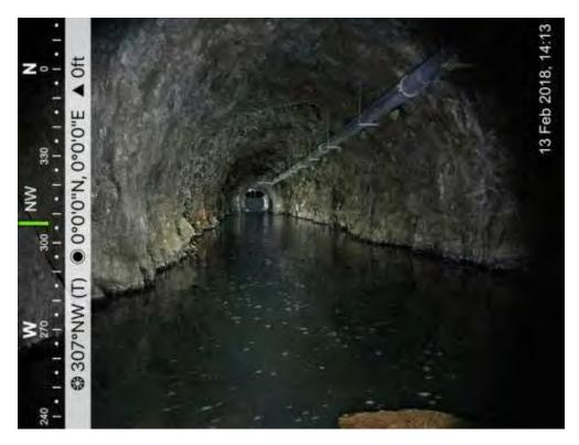
Photograph 5-6: Iron Gate Diversion Tunnel Interior Section of Unlined Rock, February 13, 2018
