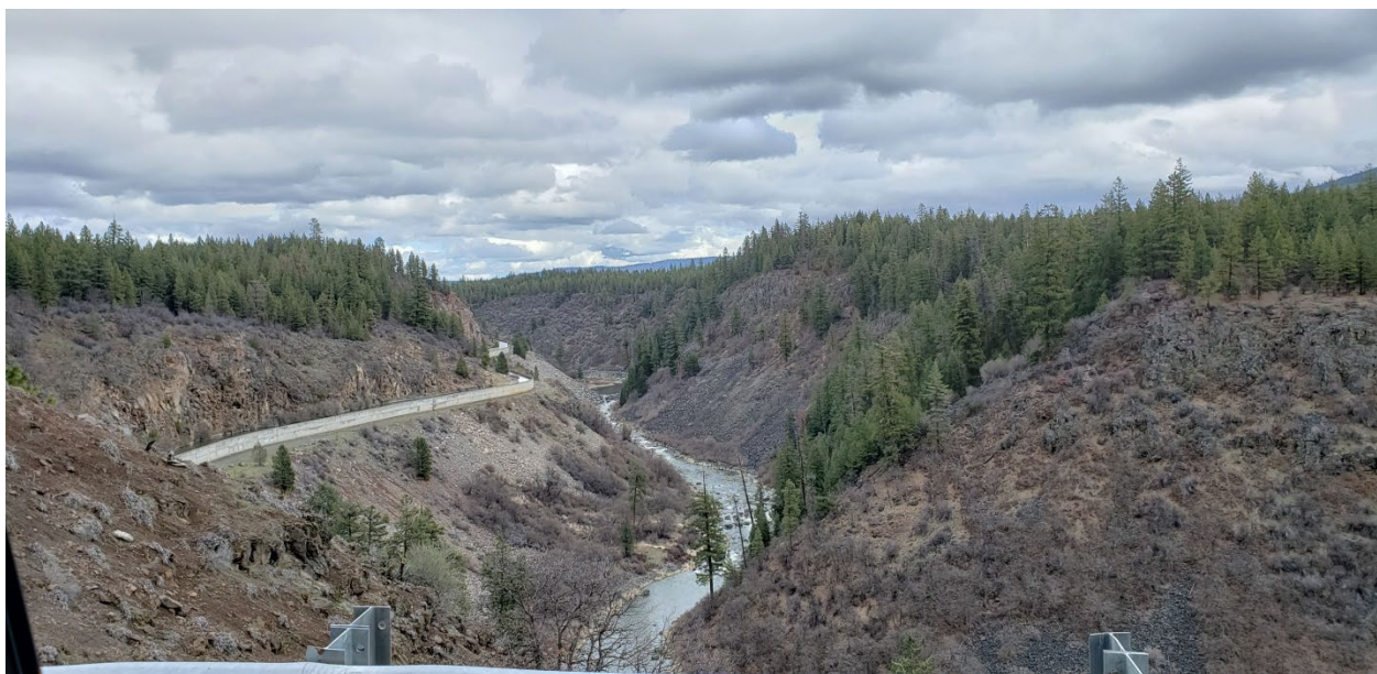
Figure 2-6: View of J.C. Boyle Bypass Reach, Klamath River Canyon and Power Canal
