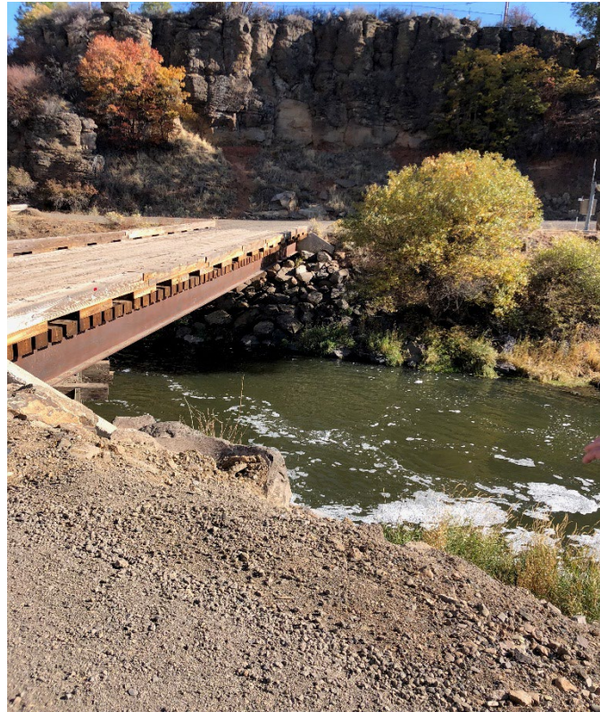
Figure A-8: Potential Moonshine Falls River Access Site – Existing Conditions at Timber Bridge
