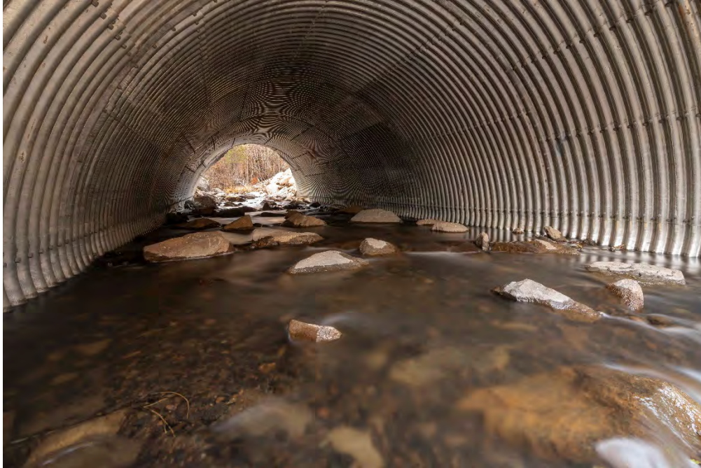
Image 2. Elder Creek Multi-plate sunken culvert 21 ft span, 13 ft rise
