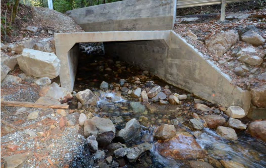
Image 4. Corrolitos Creek Sunken Box Culvert
