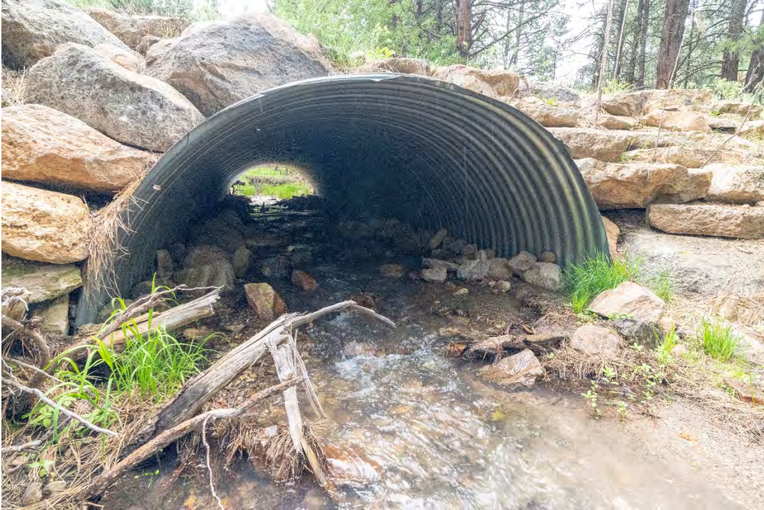
Image 6Howard Creek Tributary sunken culvert (span 12 ft, 8 ft rise)
