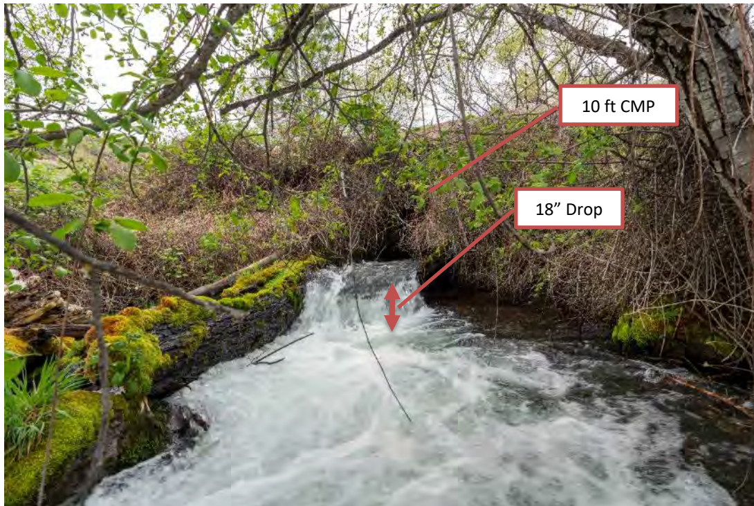
Image 4. Looking upstream at Daggett Culvert outlet
