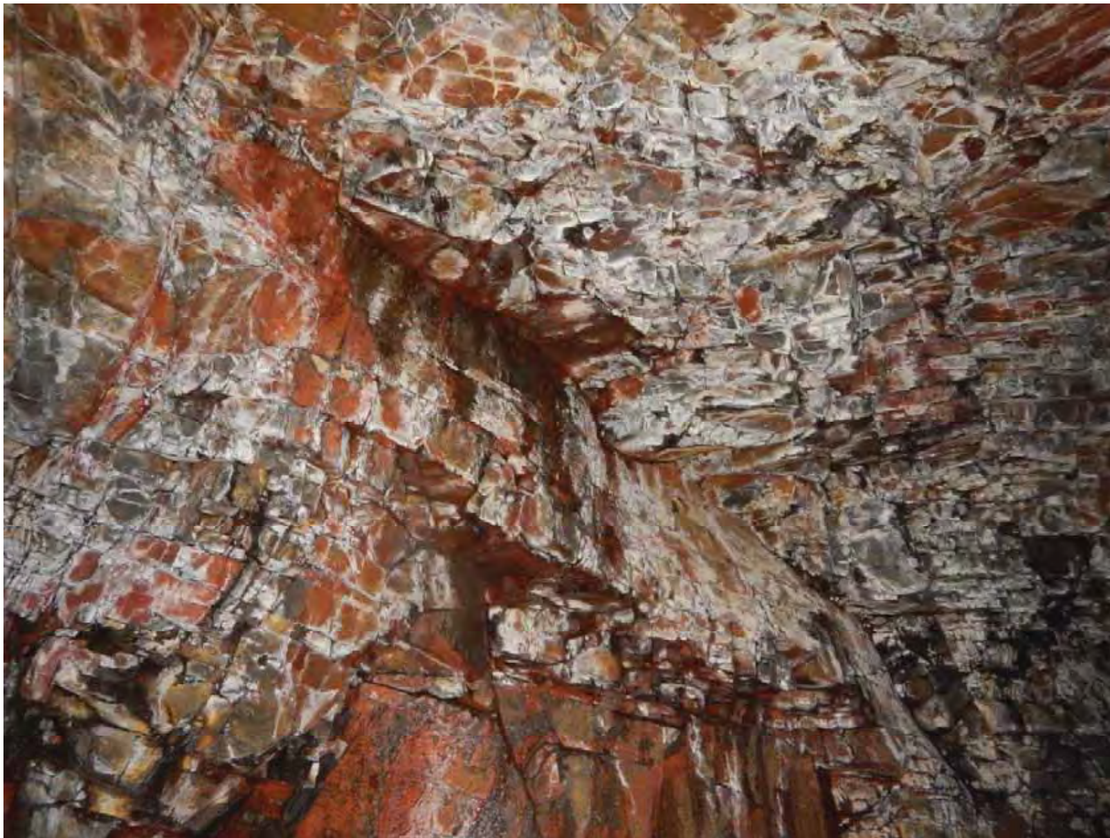
STA 453.7 ft – 9.8 ft long triangular wedge failure at crown/wall interface formed by intersection of Set 1 and Set 3 Joint. Note water seepage.
