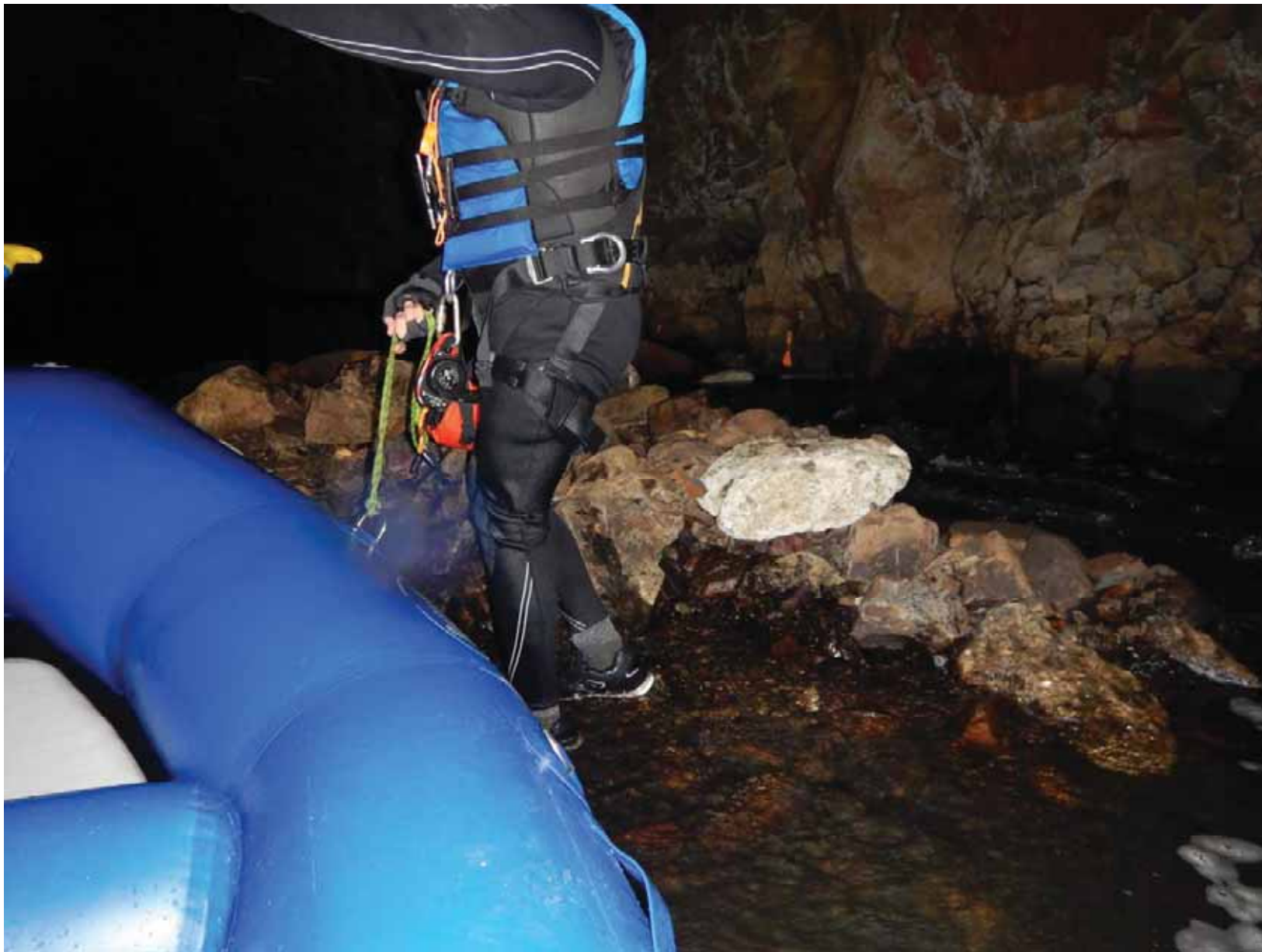
STA. 286.4 ft - 'Rubble Pile' includes concrete as well as rock fragments. No obvious evidence of a rock fall from the tunnel crown at this location
