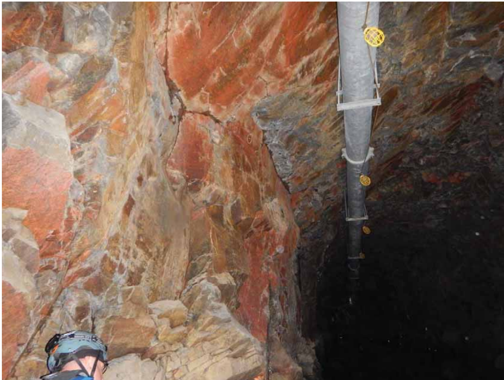
STA. 252.6 ft - Tunnel wall is developed along sub-vertical Set 1 Joint
