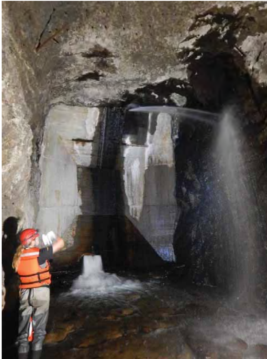
STA 176.5 ft - Tunnel Plug - Water flow at tunnel crown and seepage from top of recessed area of concrete
