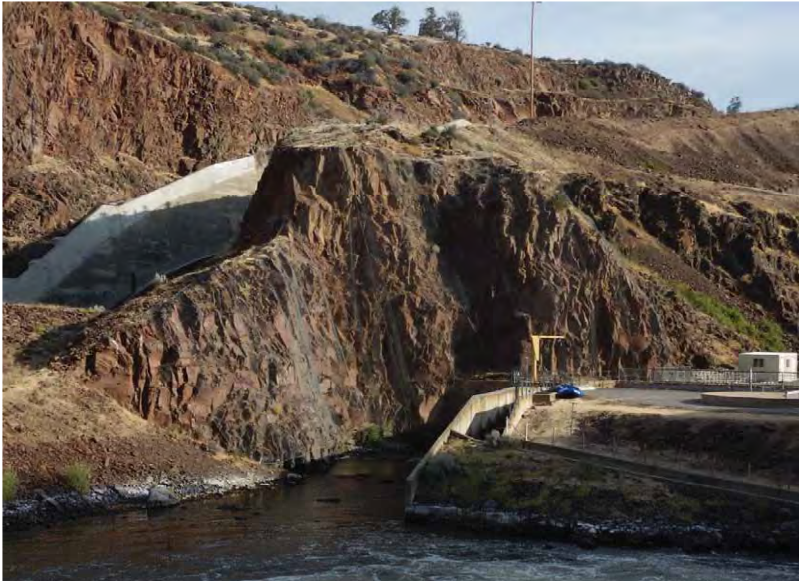
Drape Wire Mesh installed at the Downstream Portal
