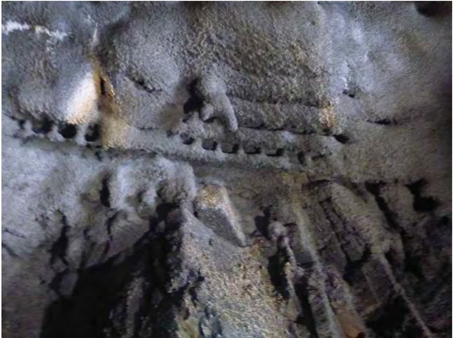
Shotcreted section with welded wire mesh and possible spot bolts
