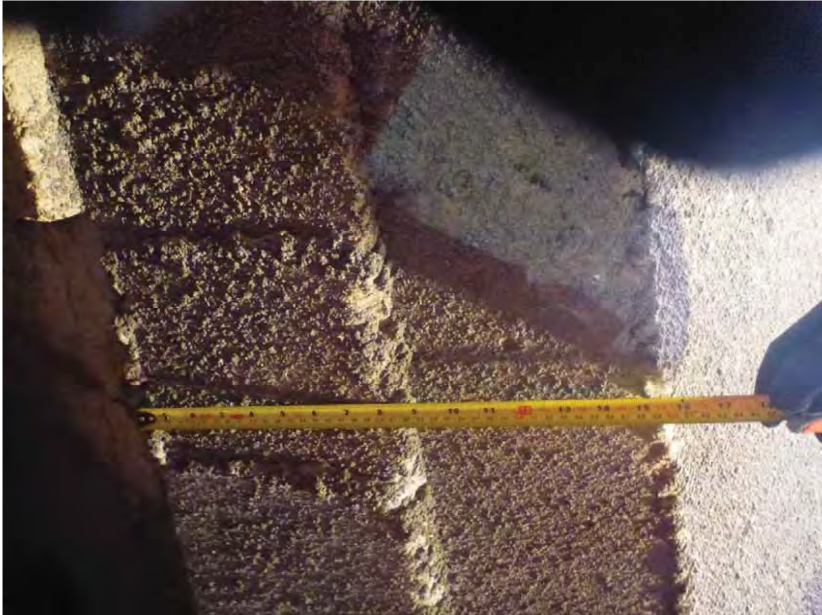
Profile of Left Wall of Downstream Concrete Liner
