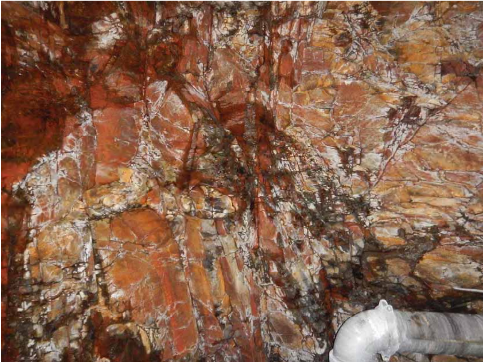
STA 509.5 ft – Seepage in Tunnel Crown
