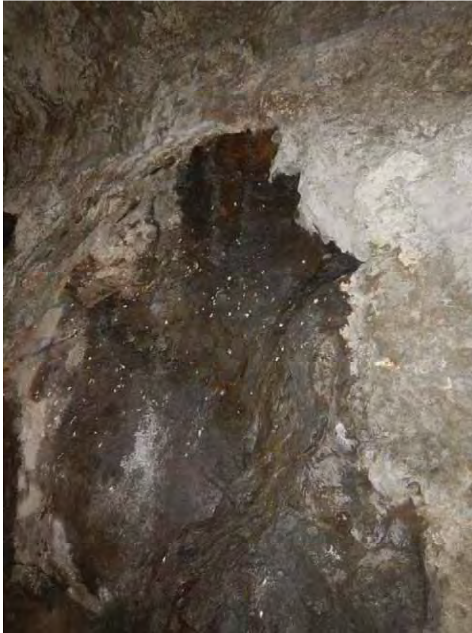
STA. 108.3 ft – Seepage from Low angle Set 3 Discontinuity
