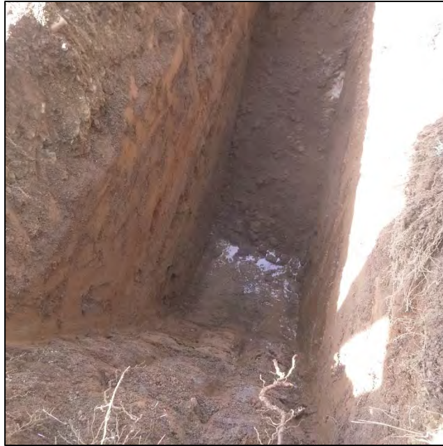
PHOTO 127 – TP-JCB-D pit excavated to depth 7.7 ft
