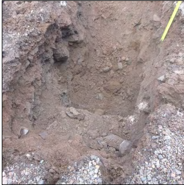
PHOTO 153 – TP-JCB-G pit excavated to depth 5.3 ft
