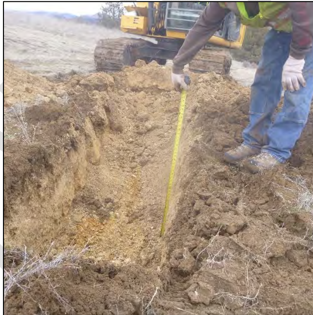
PHOTO 76 – TP-IG-D pit excavated to depth 2.3 ft
