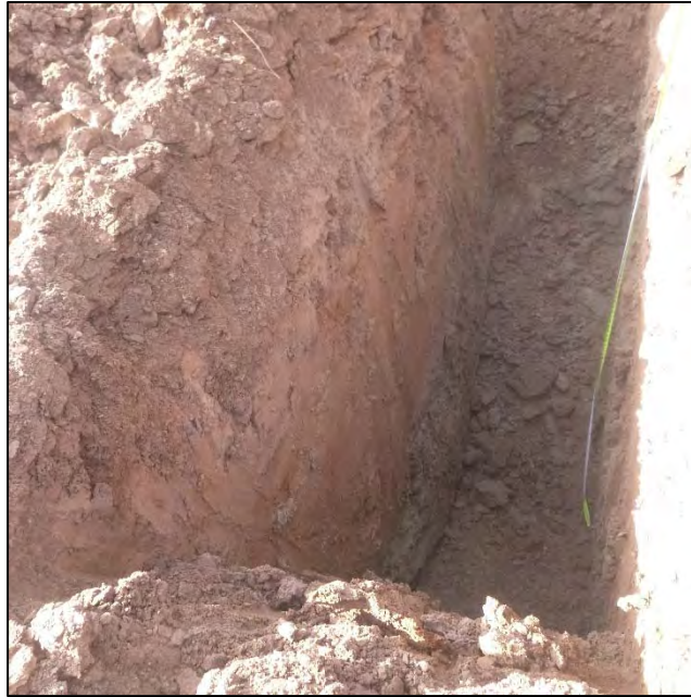
PHOTO 121 – TP-JCB-C pit excavated to depth 8.0 ft
