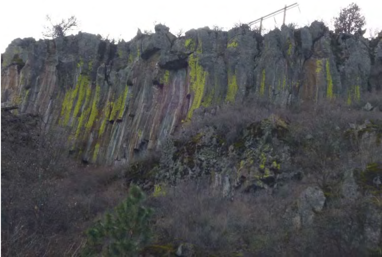
Close Up Photo of Columnar Structures and overhangs in Cliff above Left Abutment of Copco No. 2 Dam
