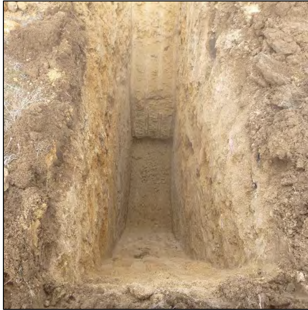
PHOTO 83 – TP-IG-D pit excavated to final depth 12.7 ft
