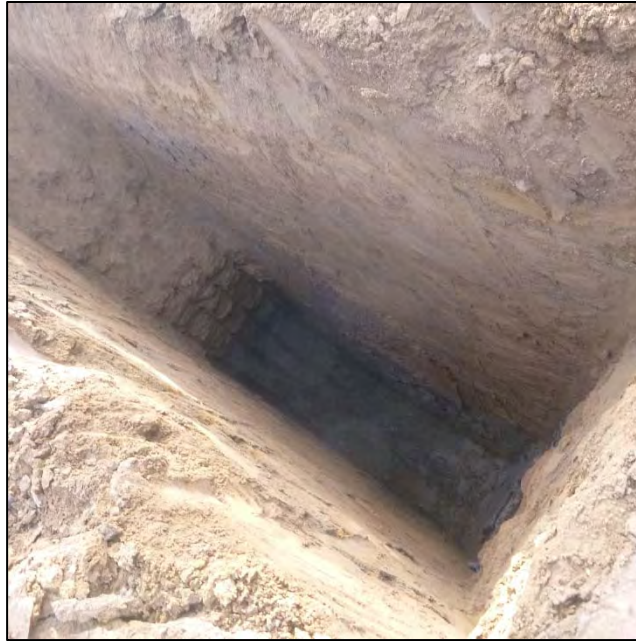
PHOTO 101 – TP-JCB- A pit excavated to depth 14.9 ft
