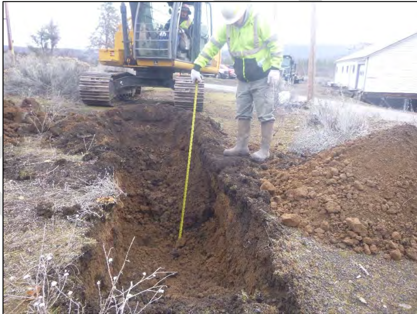
PHOTO 34 – TP-CO1-E pit excavated to depth 3.4 ft
