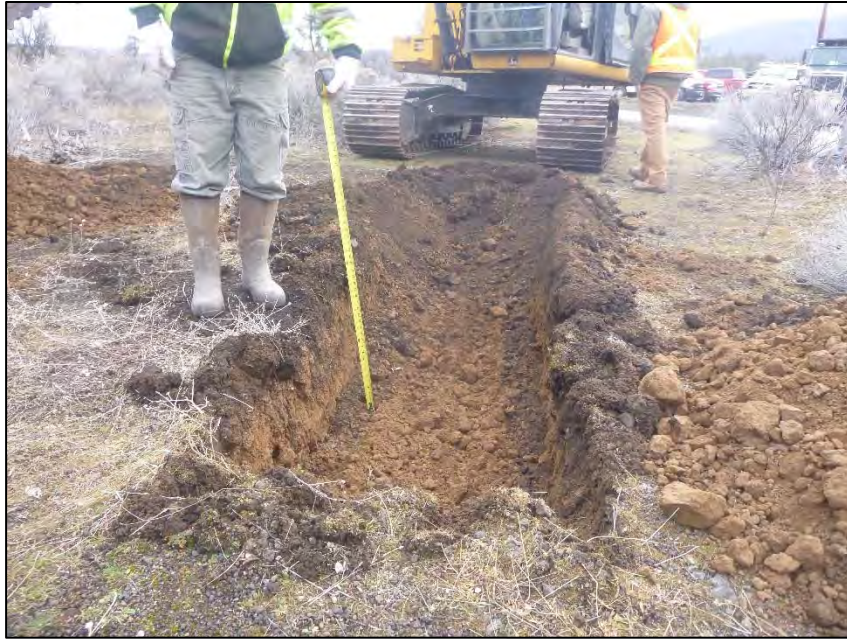
PHOTO 33 – TP-CO1-E pit excavated to depth 1.4 ft
