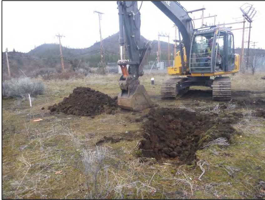
PHOTO 17 – TP-CO1-C pit excavated to depth 2.3 ft
