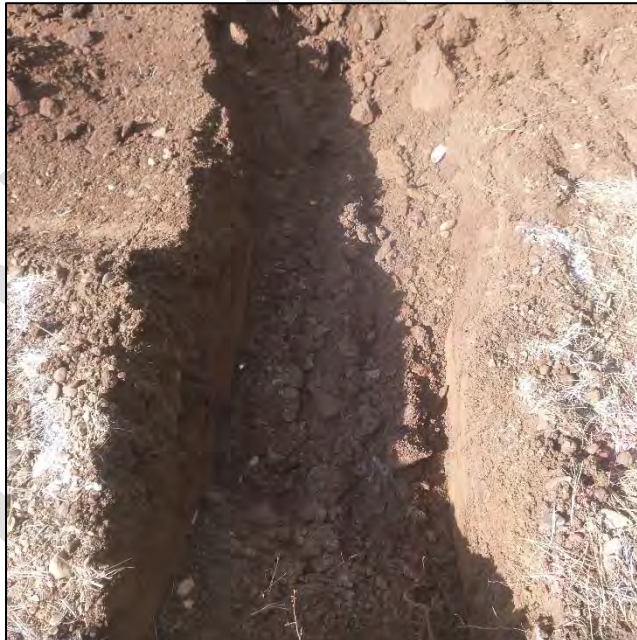
PHOTO 126 – TP-JCB-D pit excavated to depth 1.7 ft
