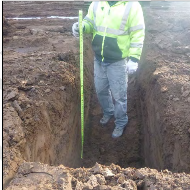
PHOTO 96 – TP-JCB-A pit excavated to depth 3 ft
