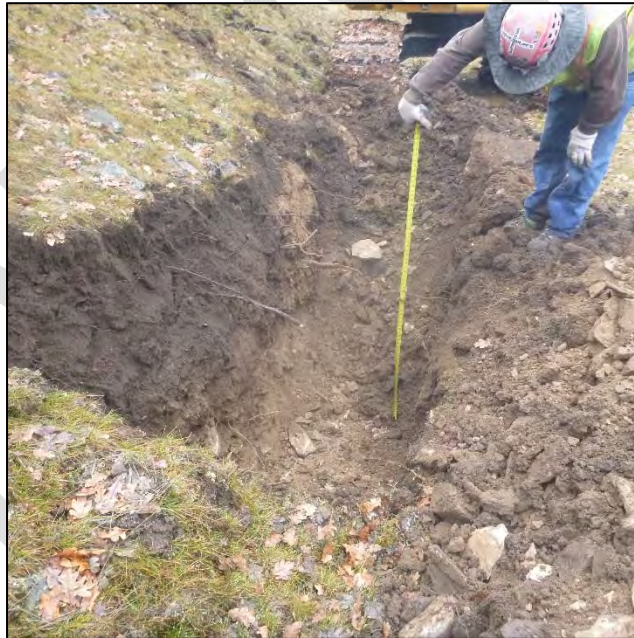
PHOTO 48 – TP-CO2-B pit excavated to depth 5.2 ft
