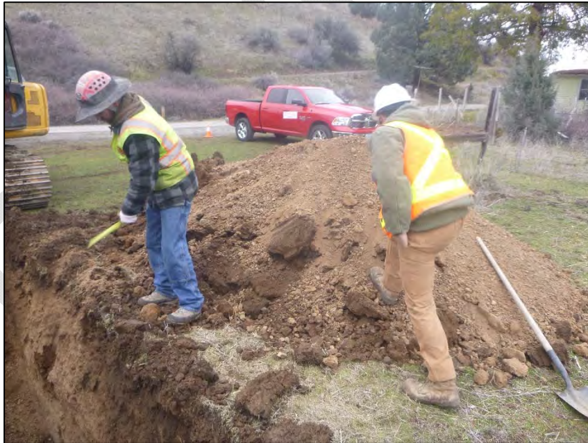
PHOTO 12 – TP-CO1-B spoils from excavation to depth 6.9 ft
