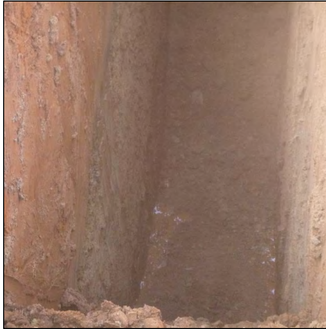
PHOTO 123 – TP-JCB-C pit excavated to depth 13.3 ft
