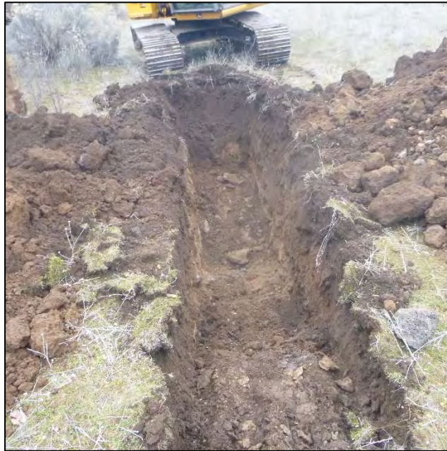
PHOTO 5 – TP-CO1-A pit excavated to final depth 6.1 ft
