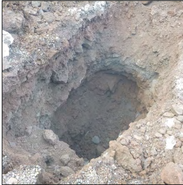
PHOTO 157 – TP-JCB-G pit excavated to depth 9.0 ft
