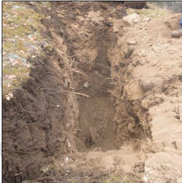
PHOTO 50 – TP-CO2-B pit excavated to final depth 11.0 ft
