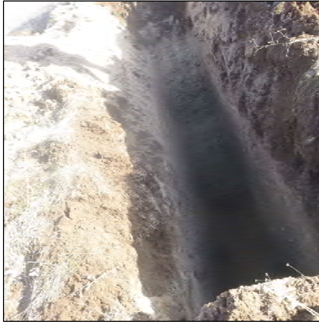
PHOTO 67 – TP-IG-B pit excavated to final depth 15.0 ft
