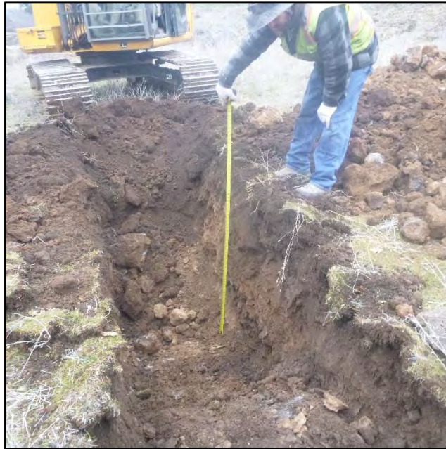
PHOTO 3 – TP-CO1-A pit excavated to depth 4.3 ft
