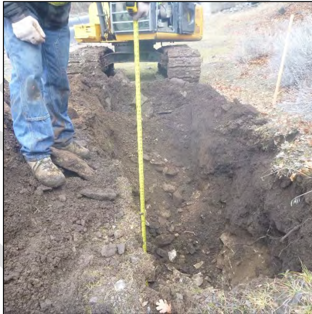
PHOTO 40 – TP-CO2-A spoils from depth 3.0 to 4.0 ft
