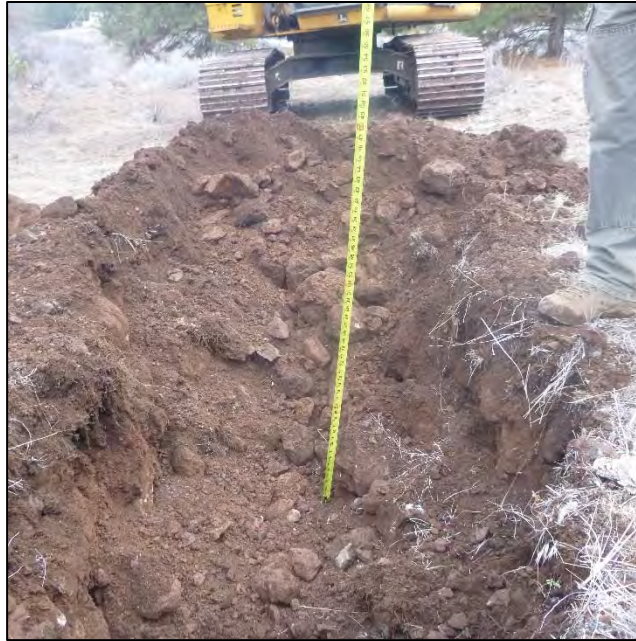
PHOTO 139 – TP-JCB-F pit excavated to depth 2.3 ft
