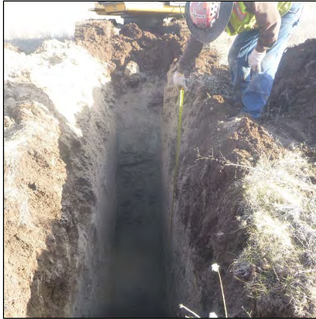
PHOTO 65 – TP-IG-B pit excavated to depth 12.0 ft
