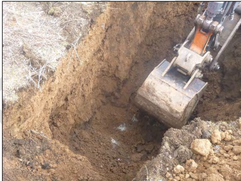
PHOTO 36 – TP-CO1-E pit excavated to final depth 8.0 ft
