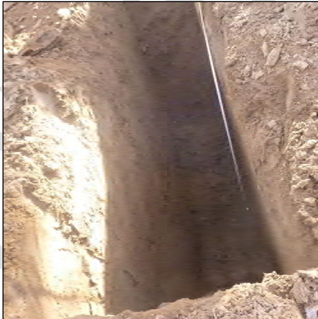
PHOTO 98 – TP-JCB-A pit excavated to depth 8.9 ft
